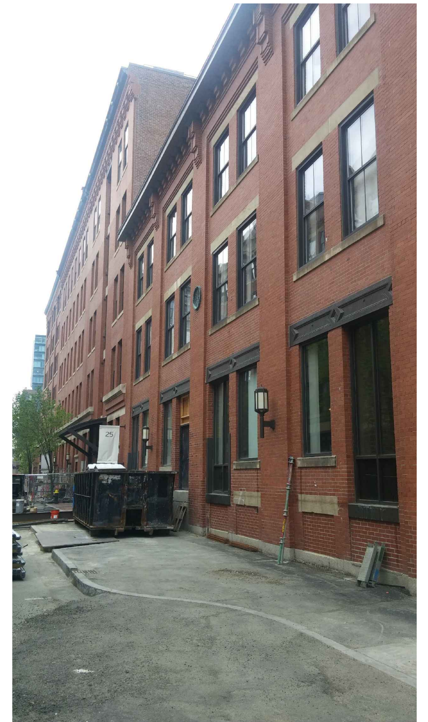
View: Looking Northeast From Thomson Place
