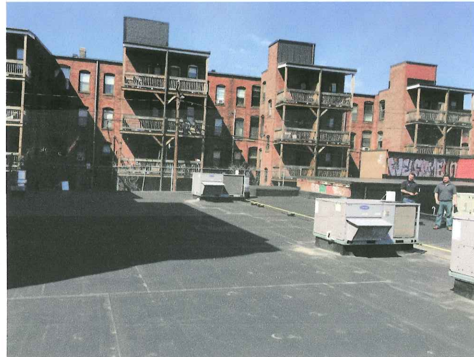
ROOFTOP LOOKING NORTH
