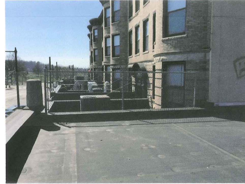
ROOFTOP LOOKING WEST
