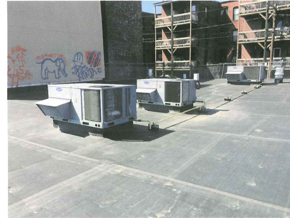
ROOFTOP LOOKING SOUTH
