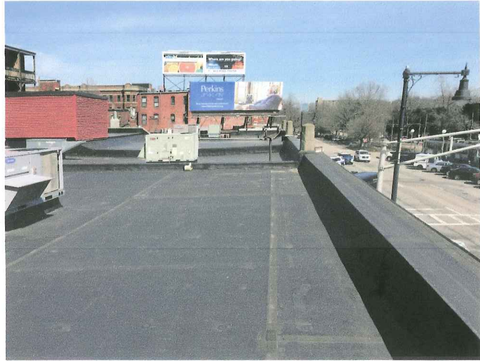
ROOFTOP LOOKING EAST
