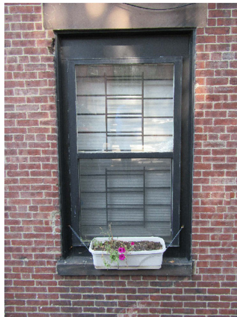
Rear Window at Lower Bay
