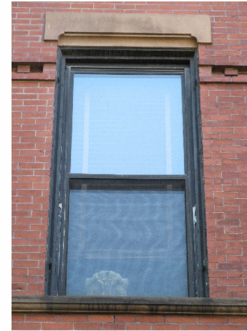
Front Window Above Entry Door
