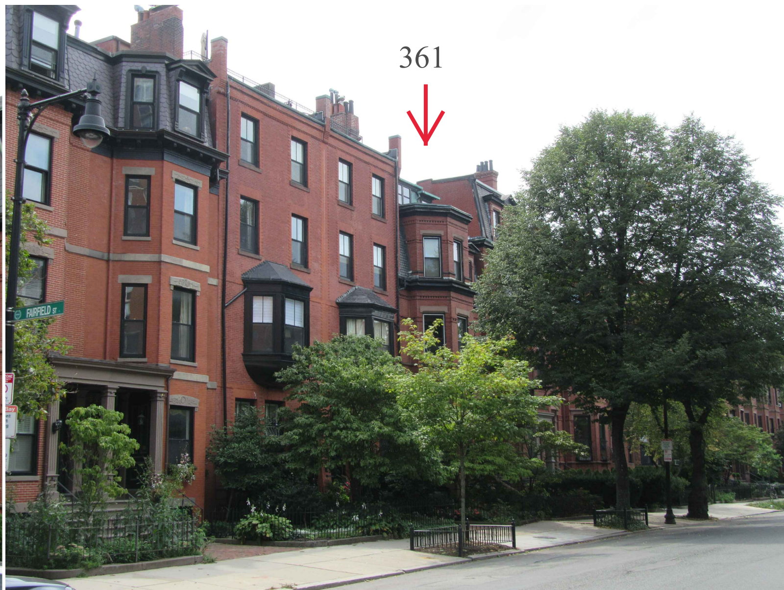
View Looking Southwest
