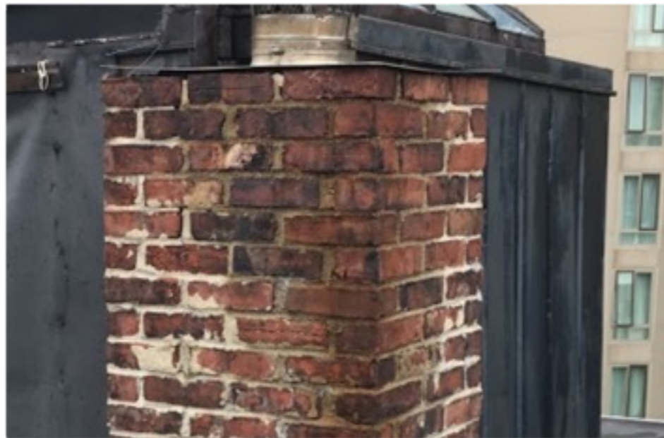
Middle Chimney Detail
