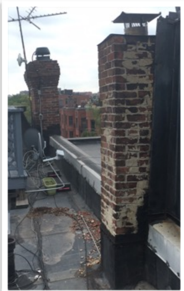
Front & Middle Chimney
