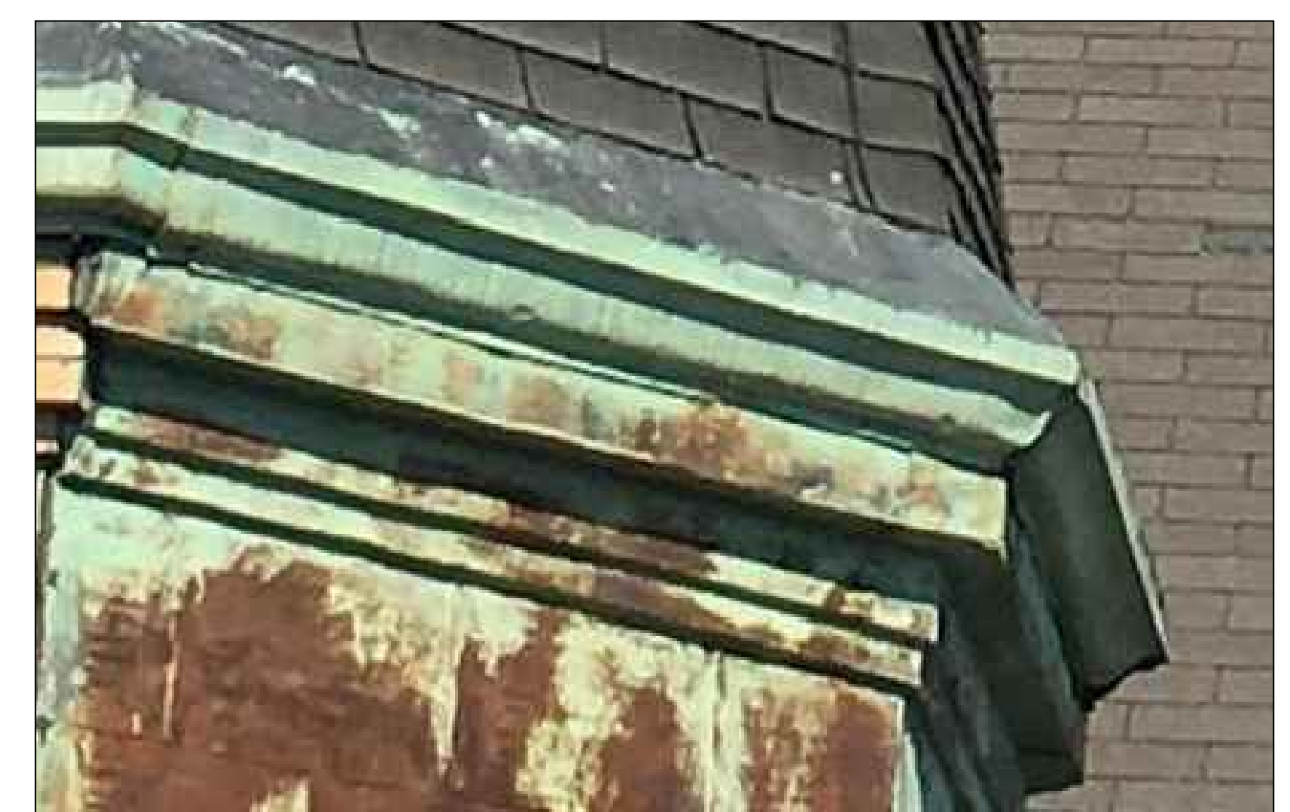
4 ROOF EAVE – TYPE 1 – PHOTO SCALE: NTS
