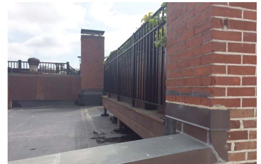
Existing Roof Decks & Penthouses Looking East
