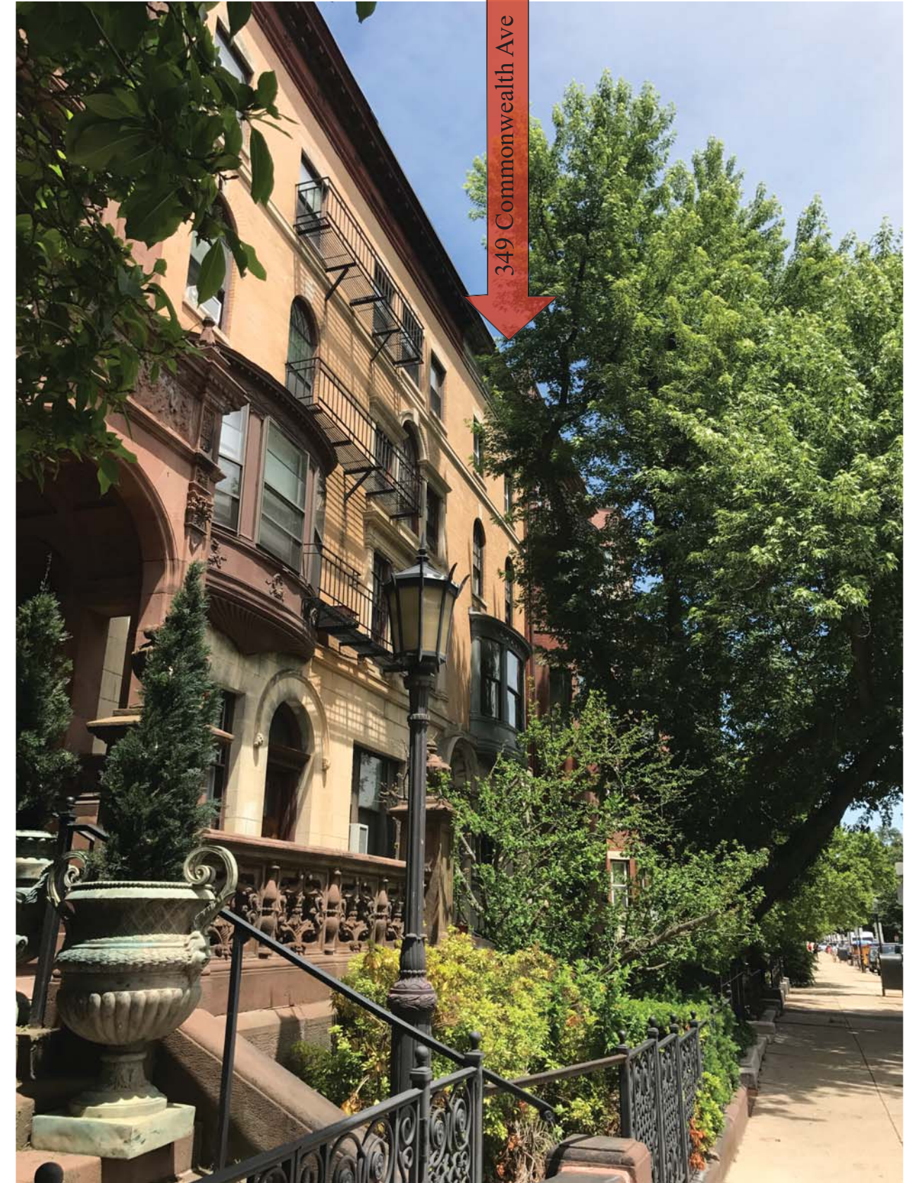
Mock-Up Looking North East on Commonwealth Ave
