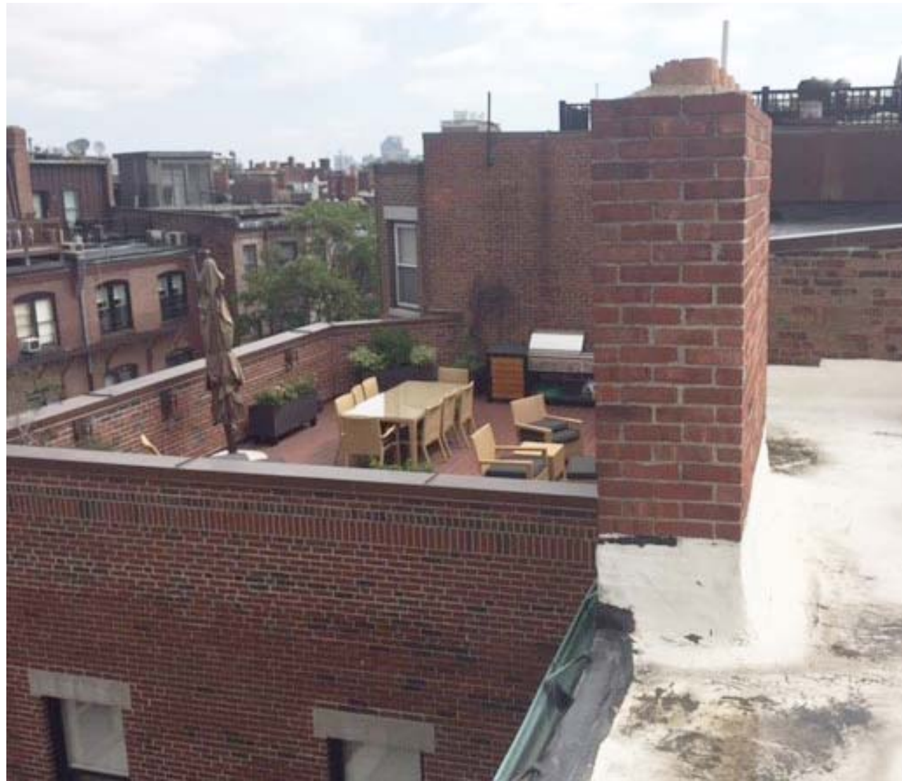
Existing Roof Decks & Penthouses Looking East
