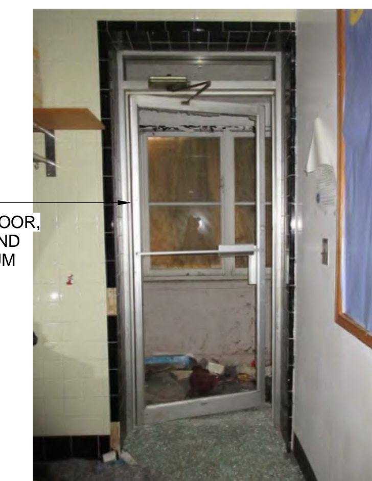
5 PHOTO NORTH COURTYARD DOOR D04
