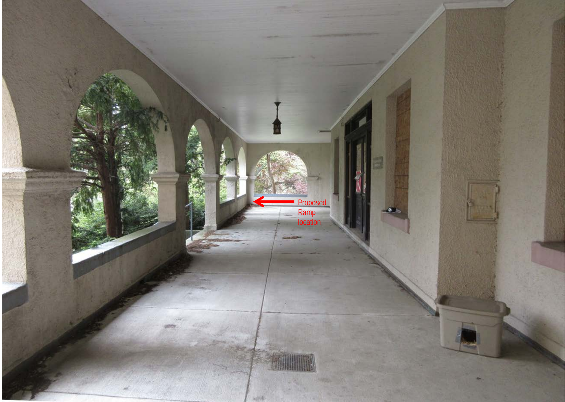
Main entry porch on east façade will be made accessible for those with physical disabilities with a new ramp concealed behind parapet wall
