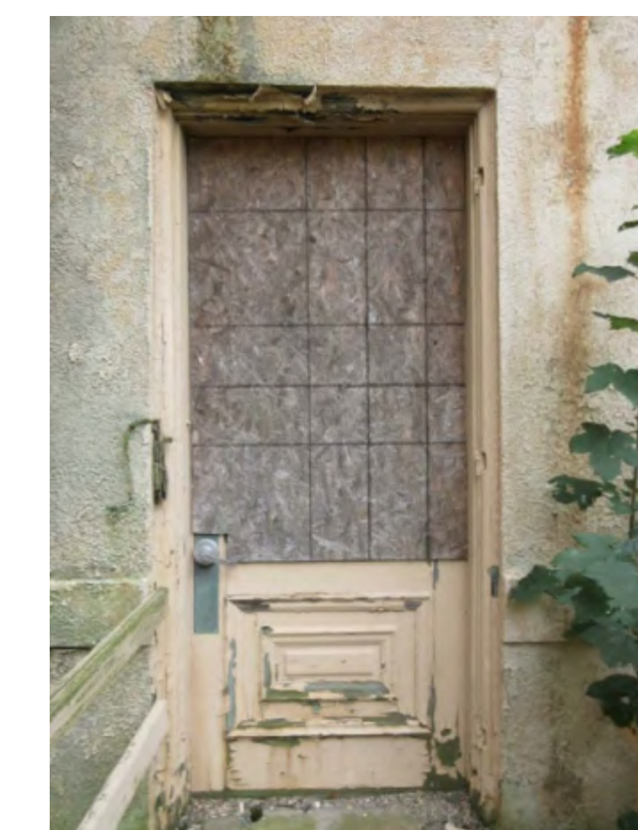
10 PHOTO AT COURTYARD DOOR D08 AT EXISTING RAMP 12" = 1'-0"
