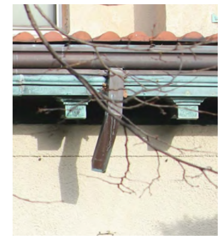
EXISTING REPLACEMENT COPPER TRIM AT PREVIOUS REPAIRS TO FRONT ENTRY PORCH, WITH MISSING DOWNSPOUT
