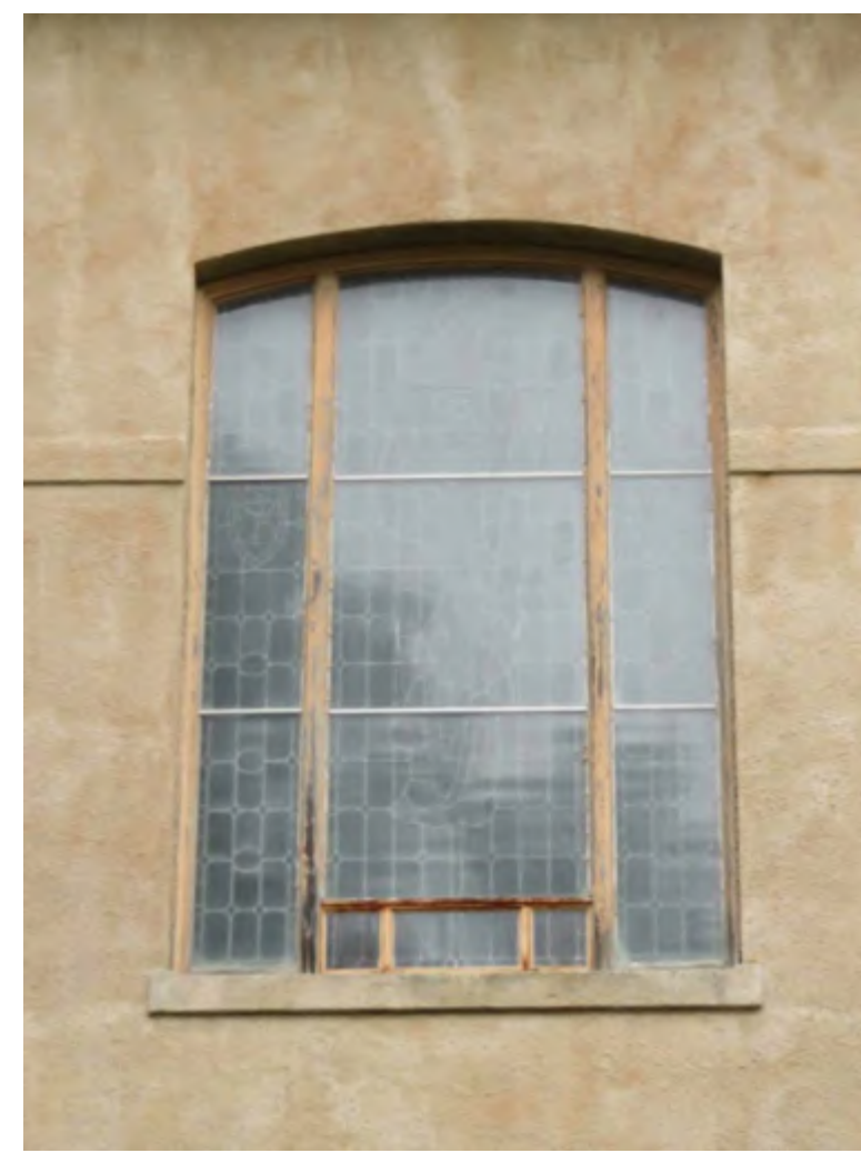
Photo showing exterior profiles of window and protective panel
