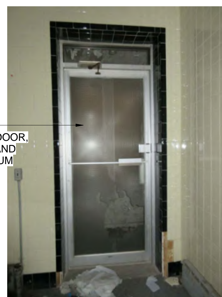
6 PHOTO AT WEST WING DOOR D05
