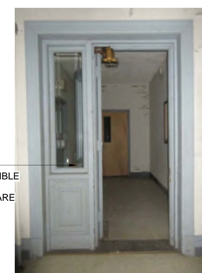
9 PHOTO AT NORTH PORCH EAST SIDE DOOR D07, INTERIOR
