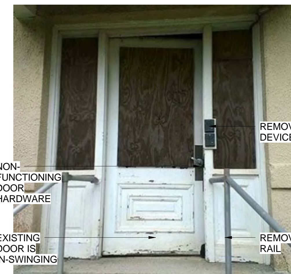
4 PHOTO CENTER COURTYARD DOOR D03
