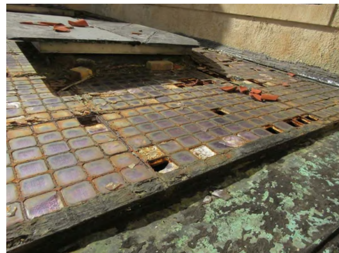
EXISTING SKYLIGHT AT COURTYARD
