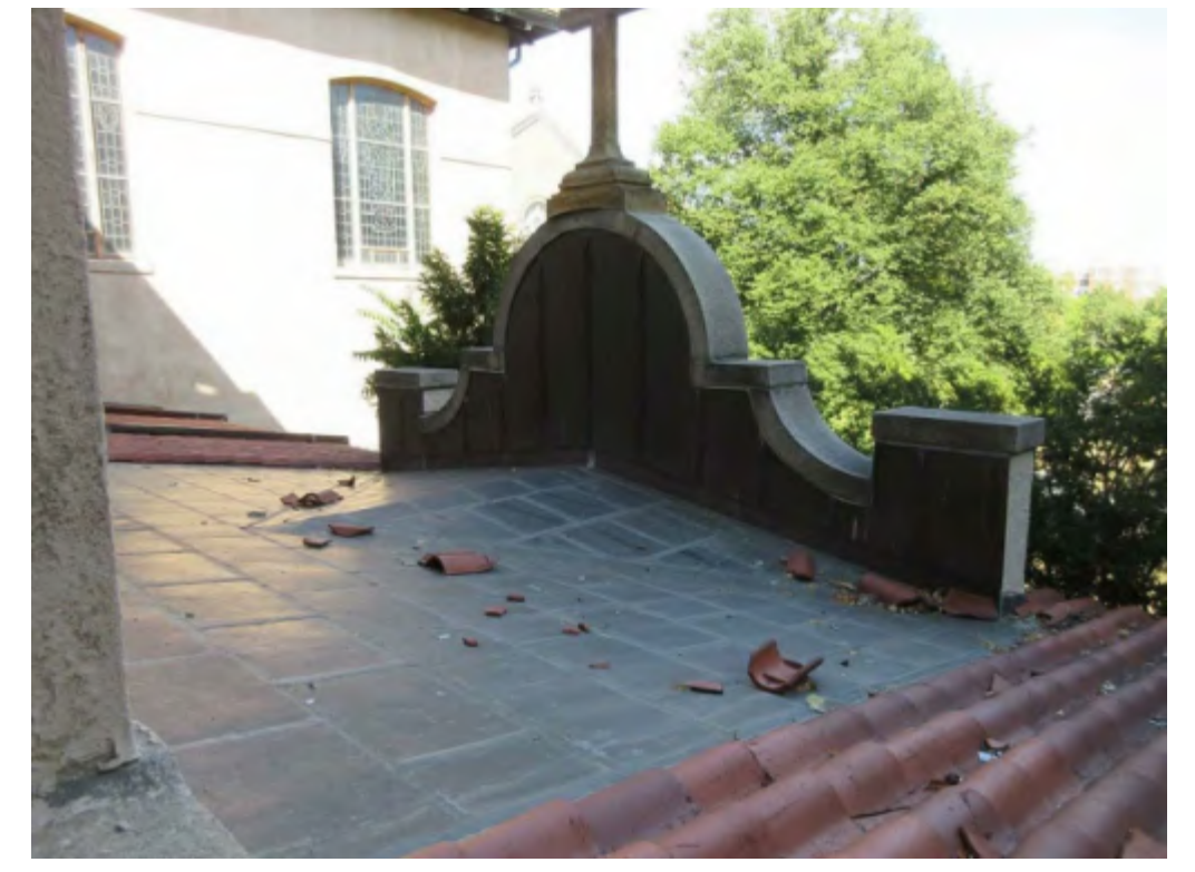
EXISTING METAL ROOF AT EAST PORCH
