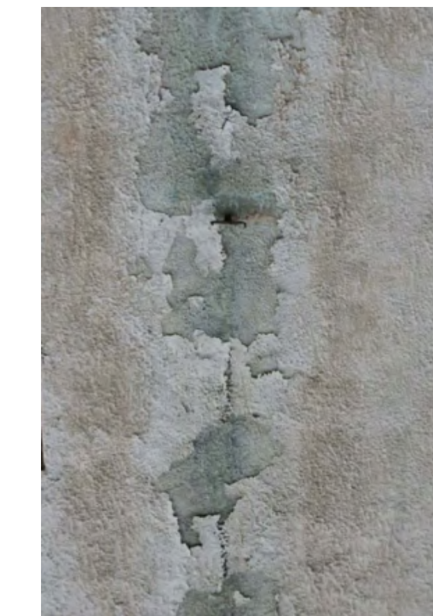
THE INTENT WILL BE TO RE-COAT TO PROVIDE UNIFORM APPEARANCE.
