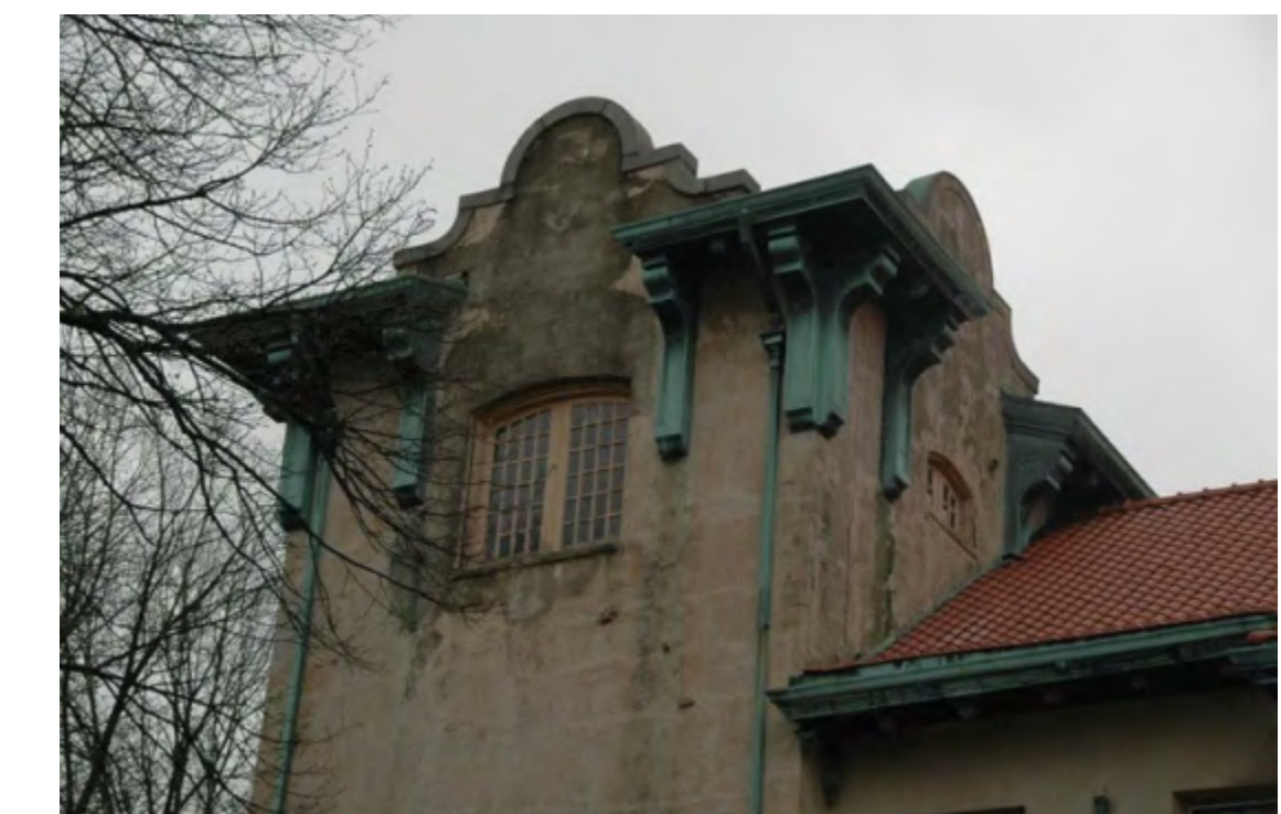
EXISTING COPPER BRACKETS, CORNICE, AND GUTTERS CAN LIKELY BE RETAINED.
