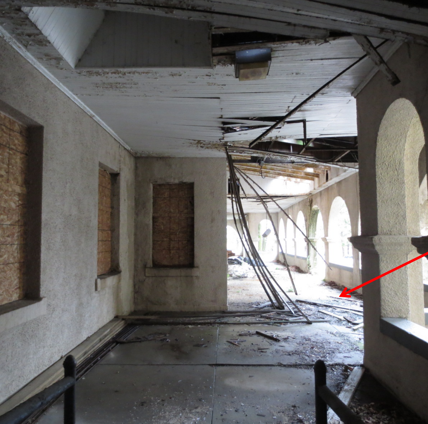
Interior of north porch to be restored due to massive damage caused by water infiltration. Accessible ramp to be concealed in porch at right side of incase.
