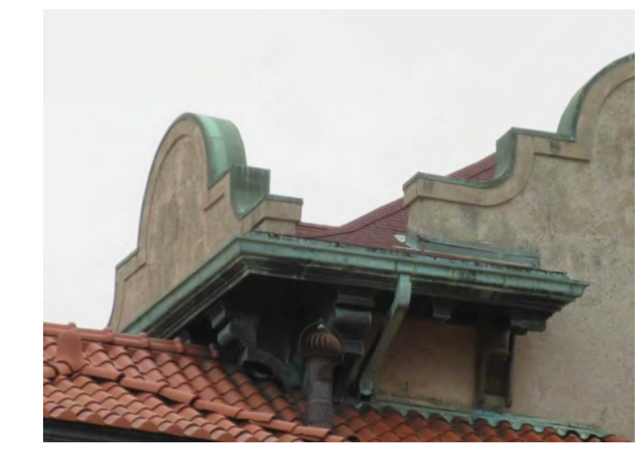
EXISTING ASPHALT SHINGLES AT TOWER ROOF
