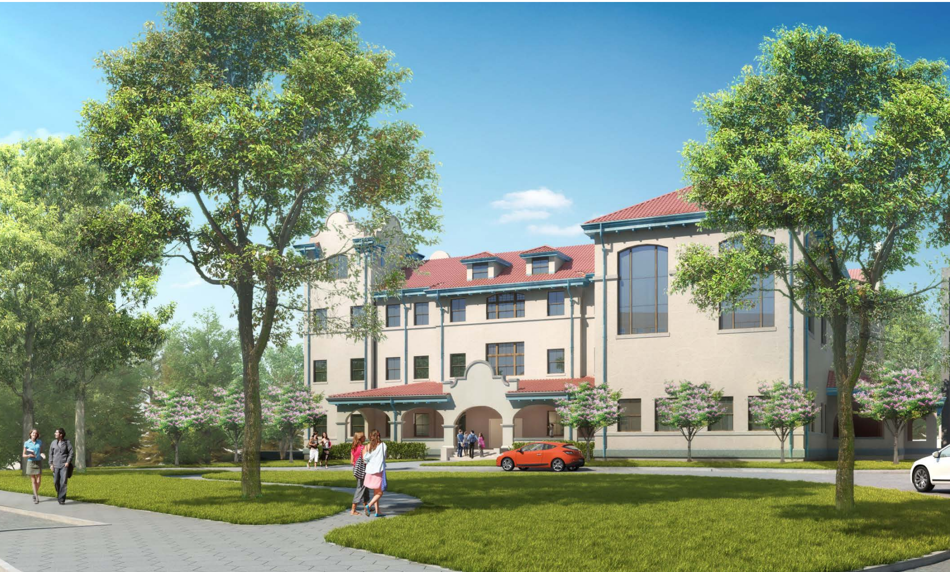
Perspective of entry of building.
