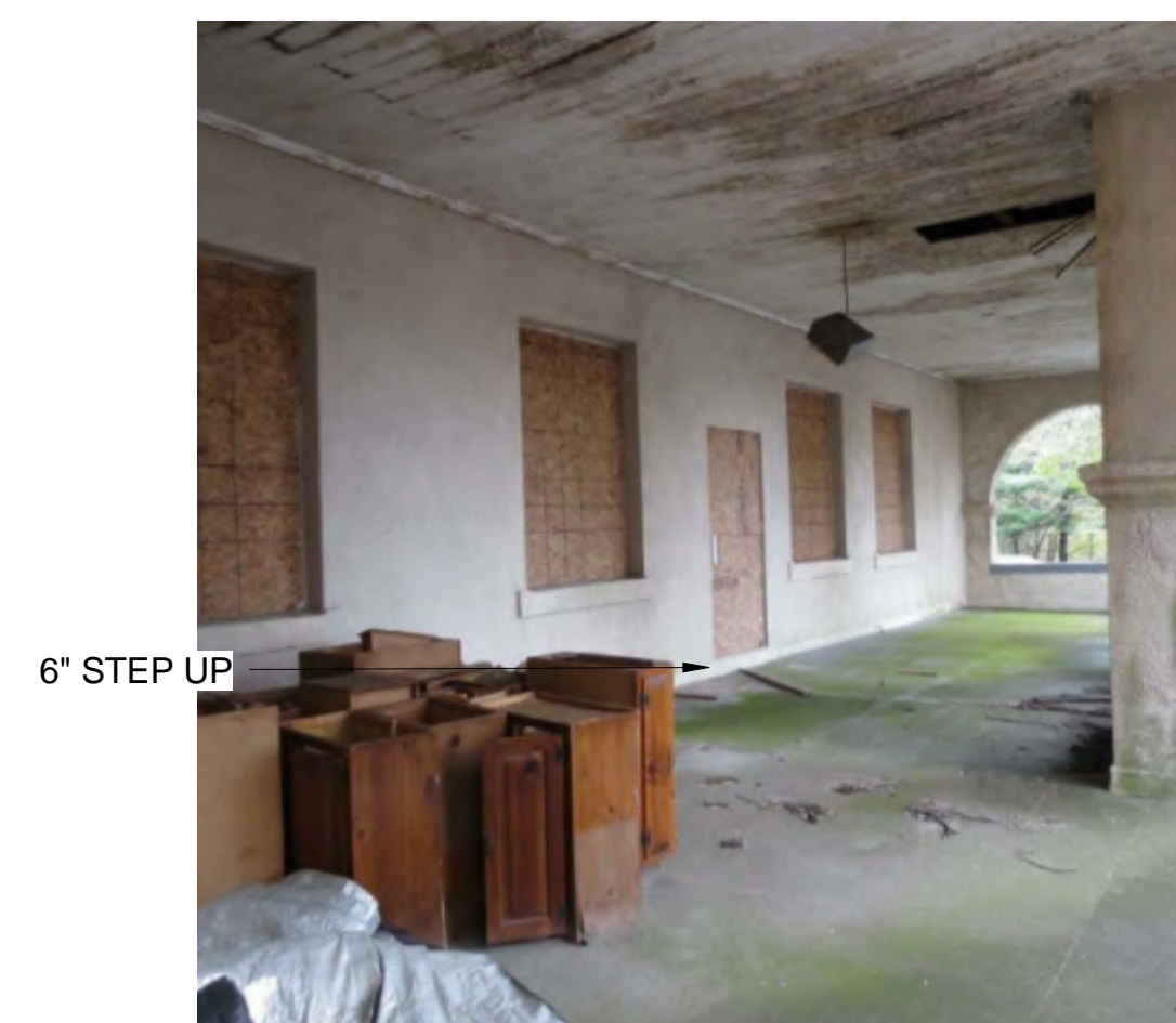
8 PHOTO AT NORTH PORCH WEST WING DOOR D06, EXTERIOR
