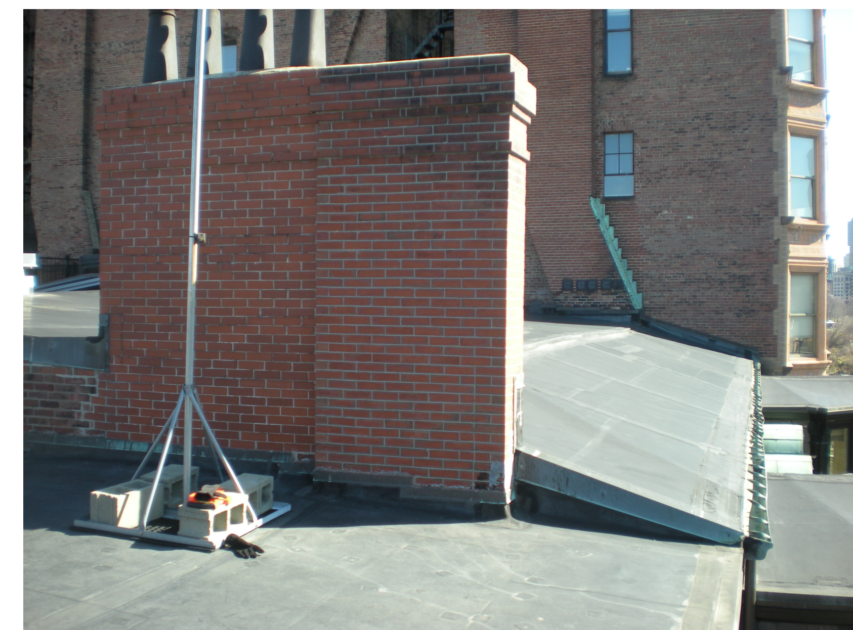
VIEW EAST TOWARD 33
