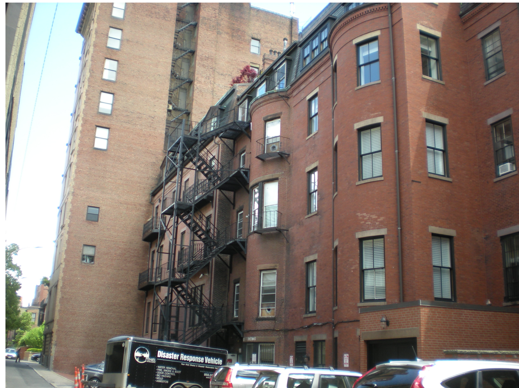
REAR FACADE LOOKING EAST
