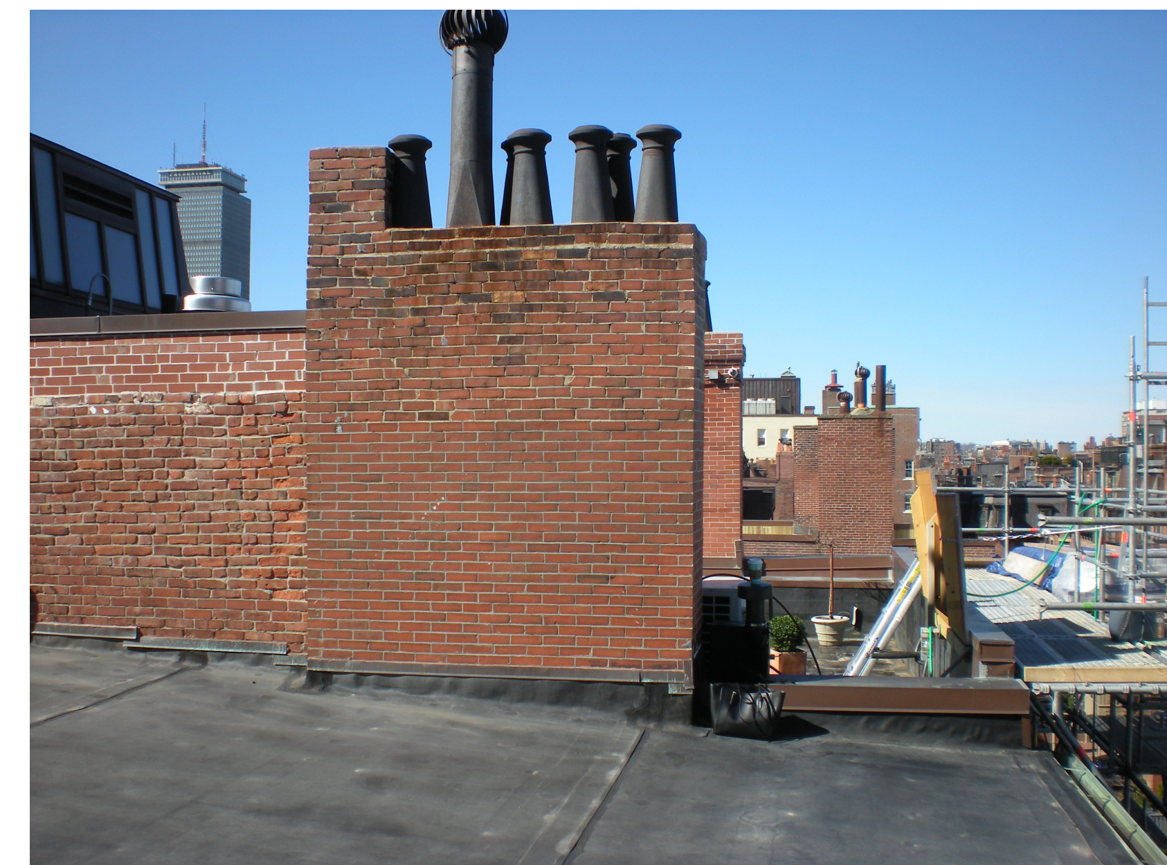
VIEW WEST TOWARD 37
