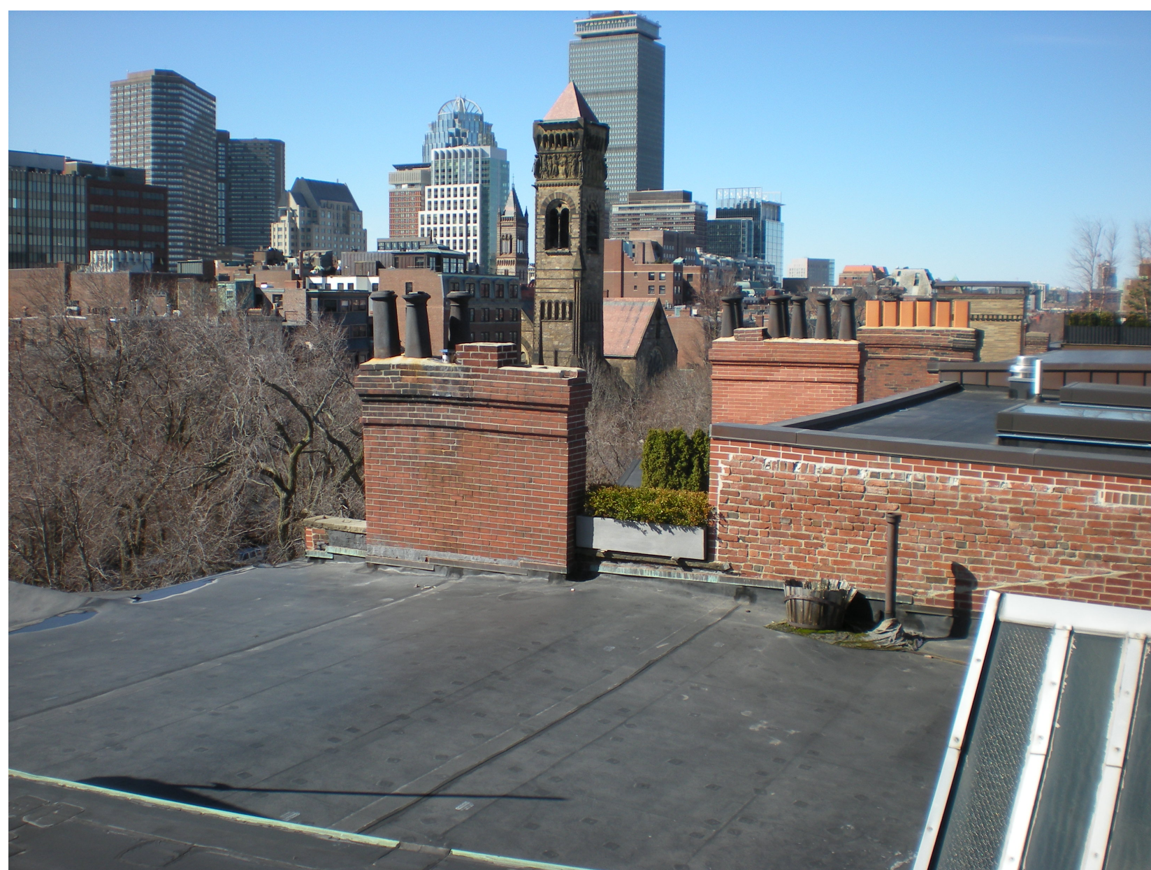
VIEW SOUTH WEST TOWARD 37
