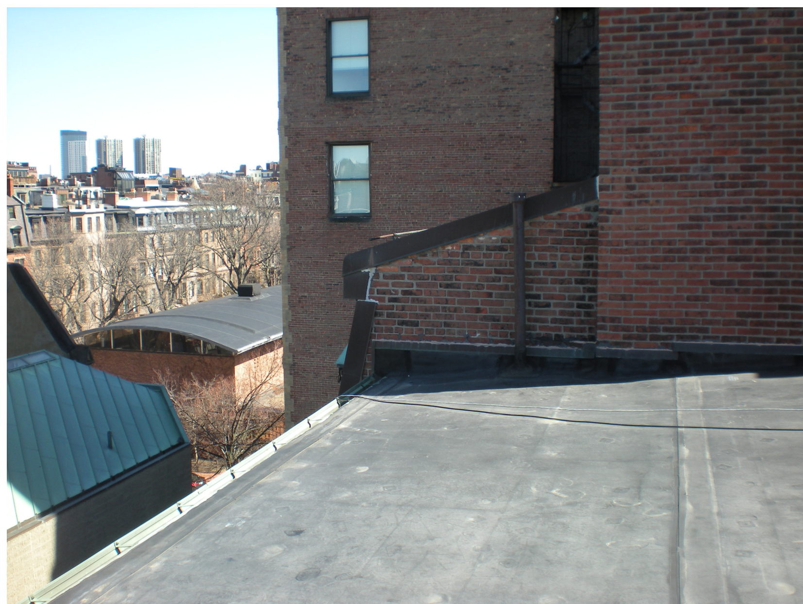
VIEW EAST TOWARD 33
