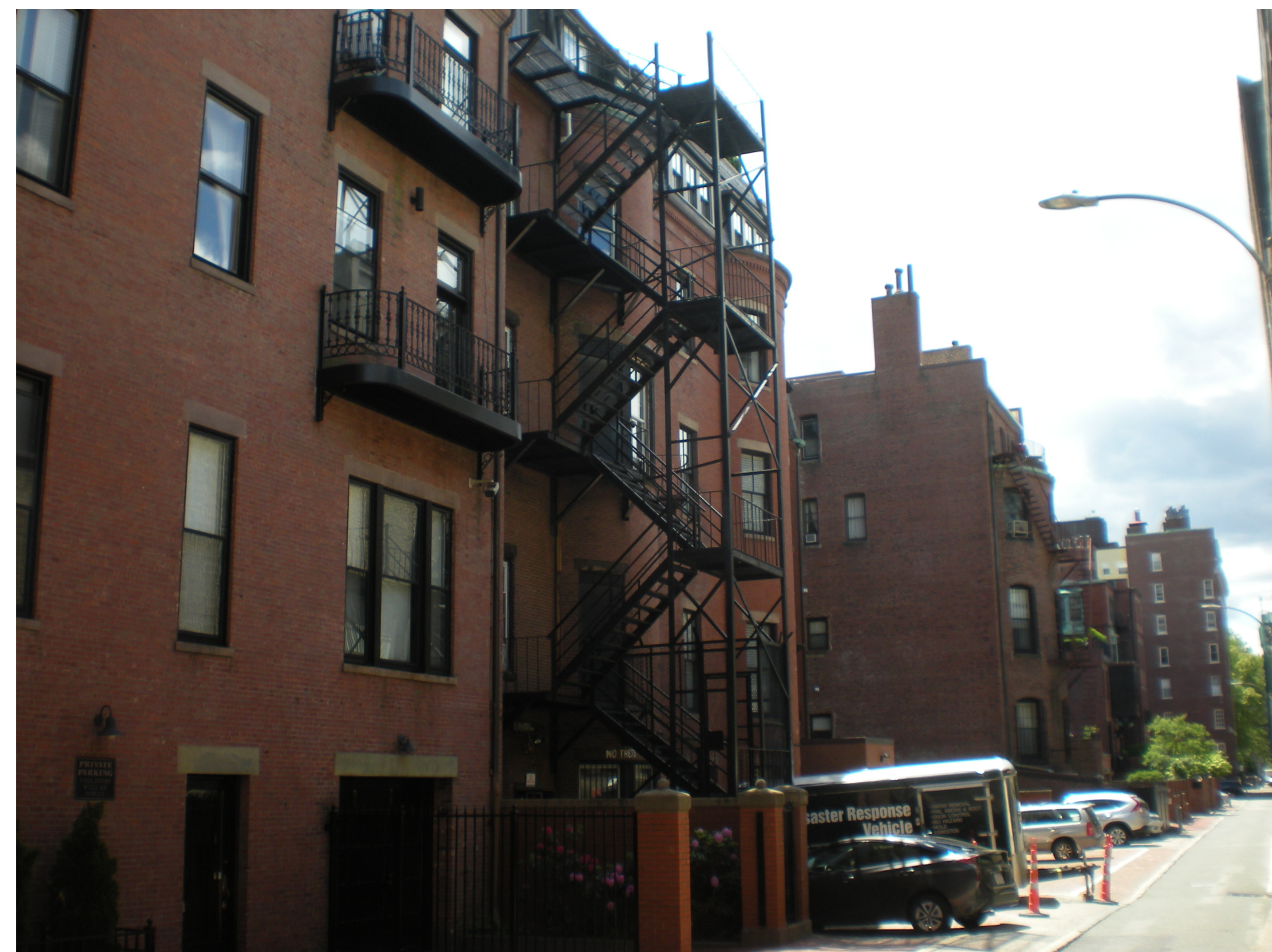
REAR FACADE LOOKING WEST
