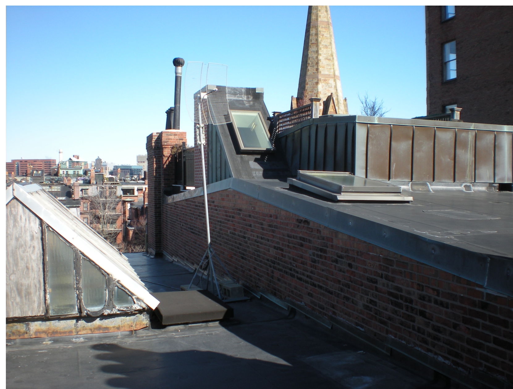
VIEW NORTH EAST TOWARD 33
