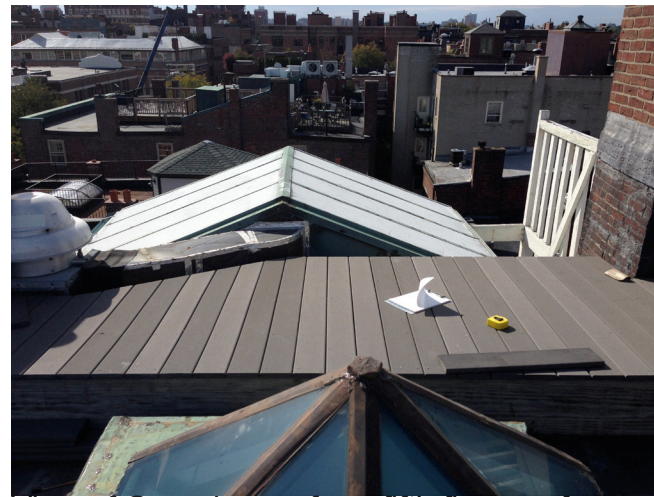
View of Greenhouse from fifth floor roof
