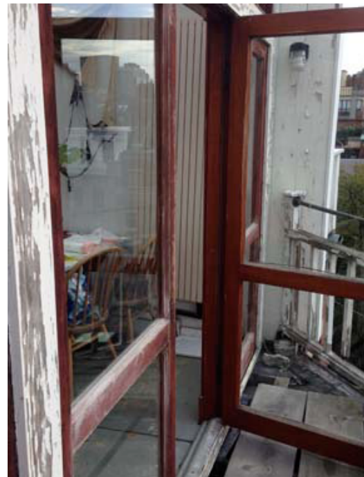
Door into Greenhouse looking towards 34 River Street party wall
