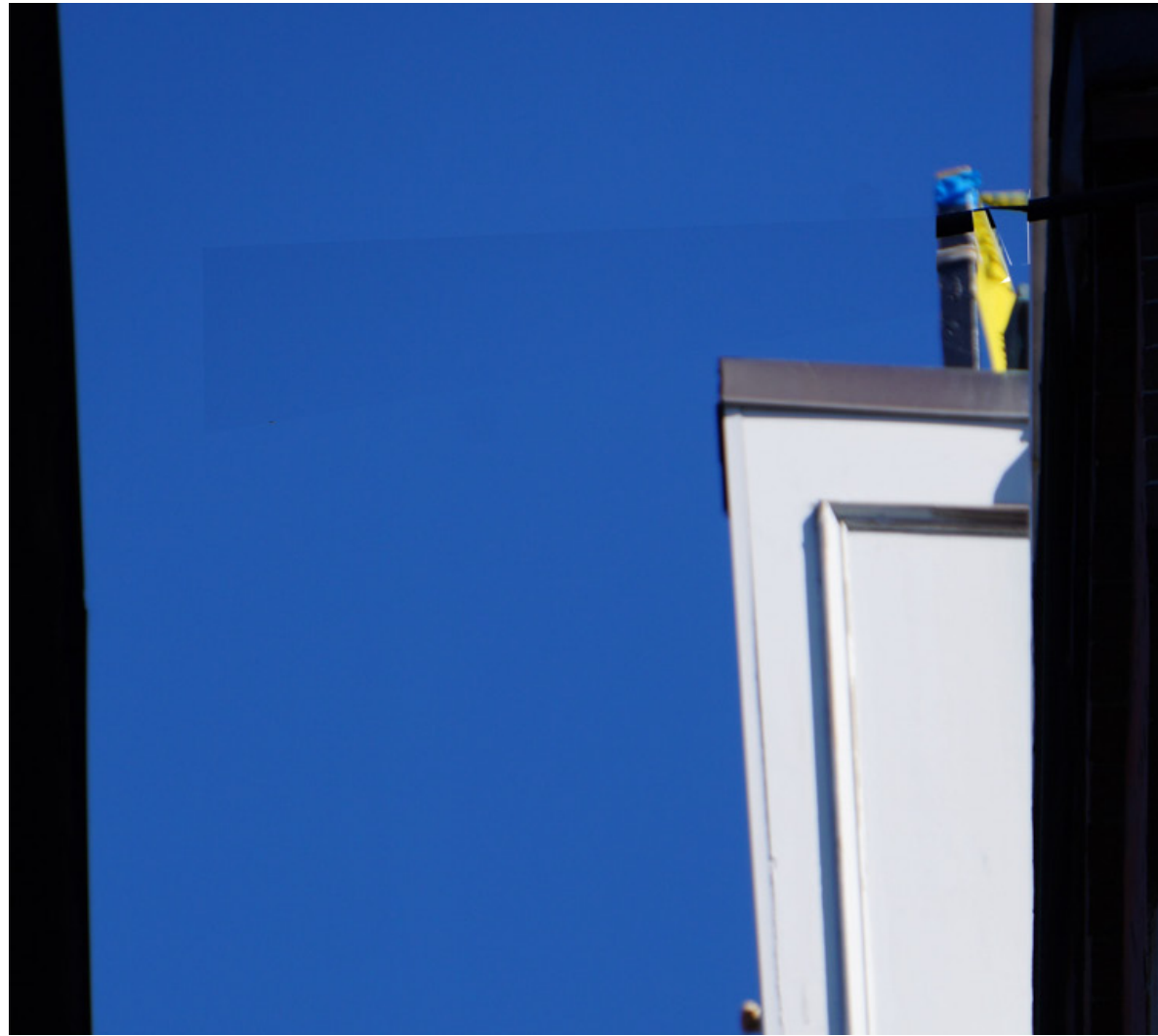
Close up of top of proposed structure, south/west corner. Yellow tape indicates location of west facade. Not visible from a public way
