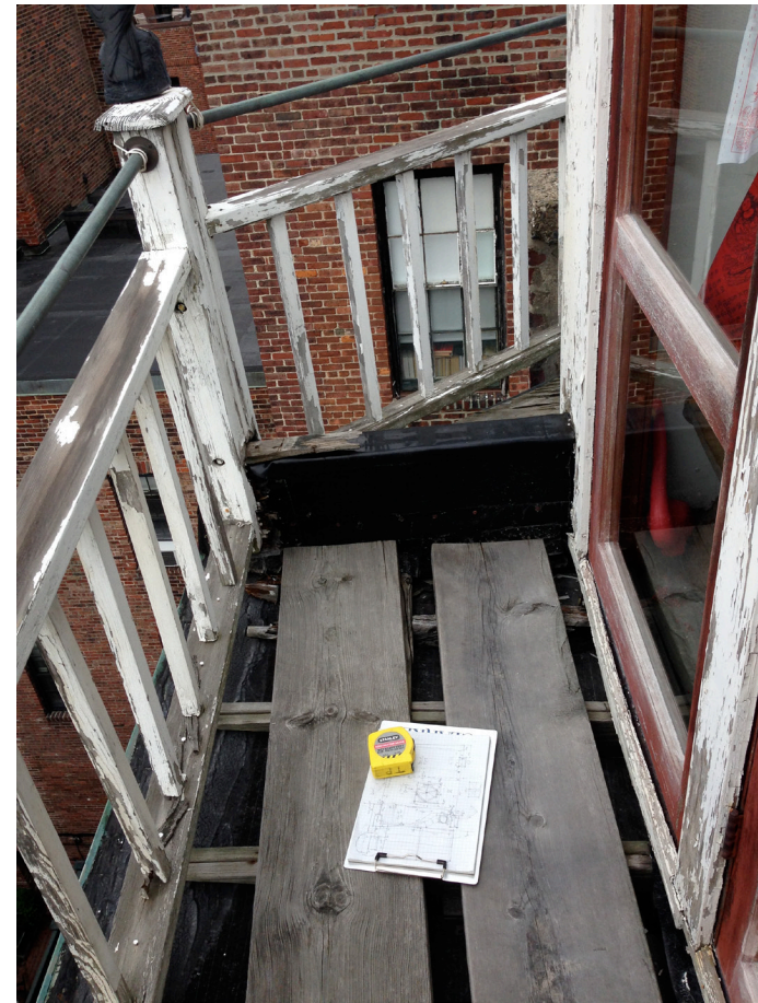
Rear Deck with exterior surface Beam
