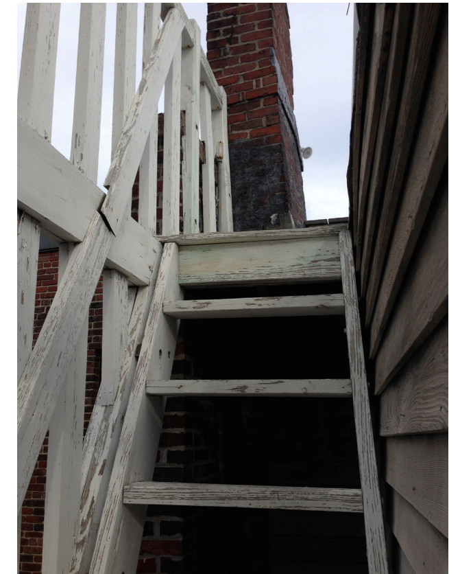
Exterior stair to Roof
