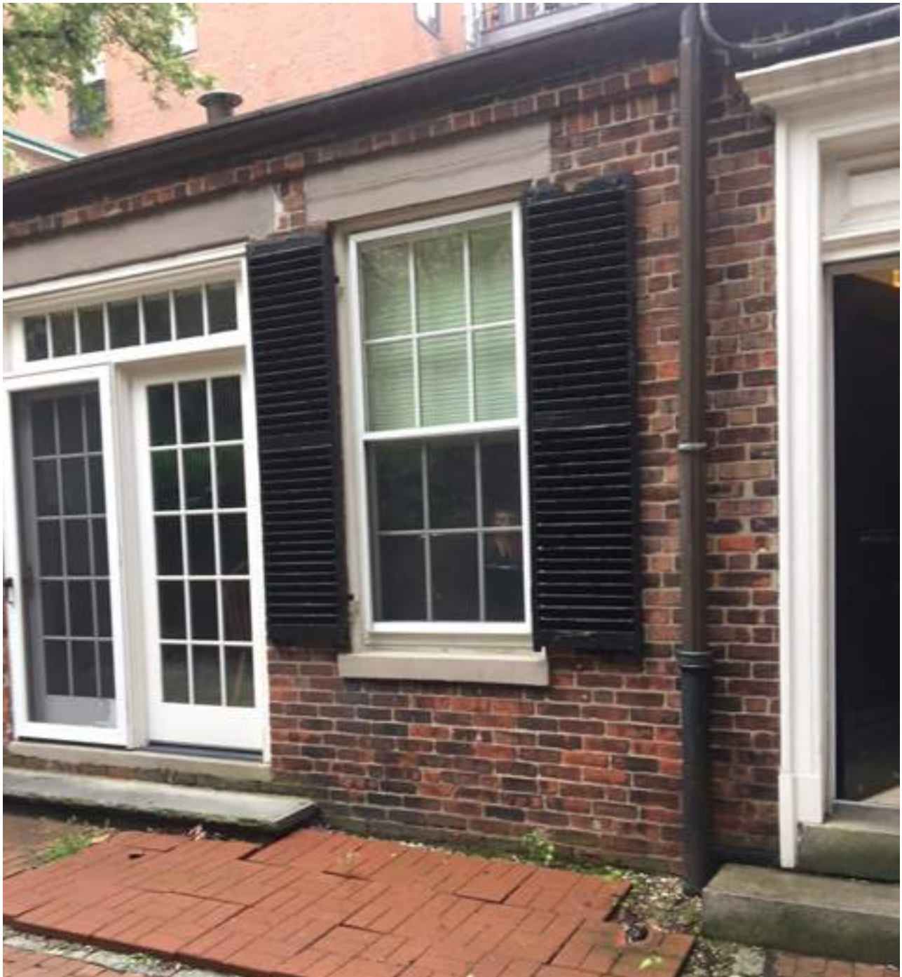
REAR SHUTTERS TO BE REMOVED
