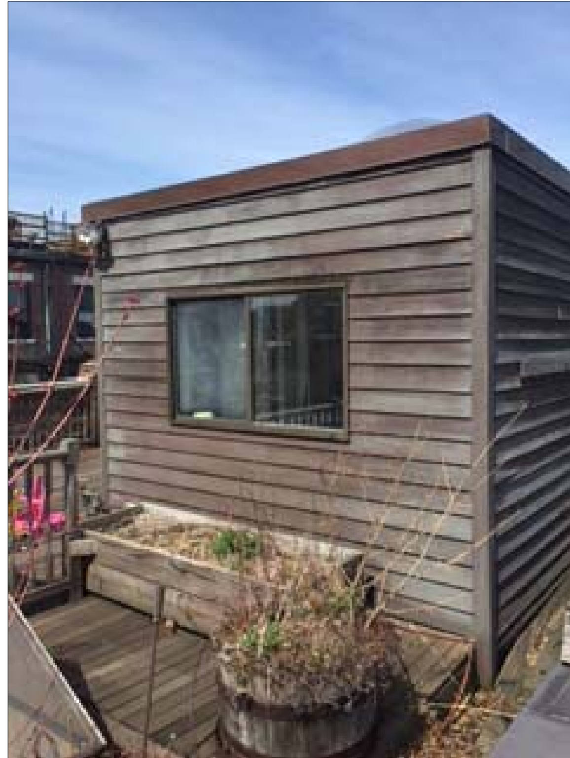
327 COMMONWEALTH AVENUE HEADHOUSE
