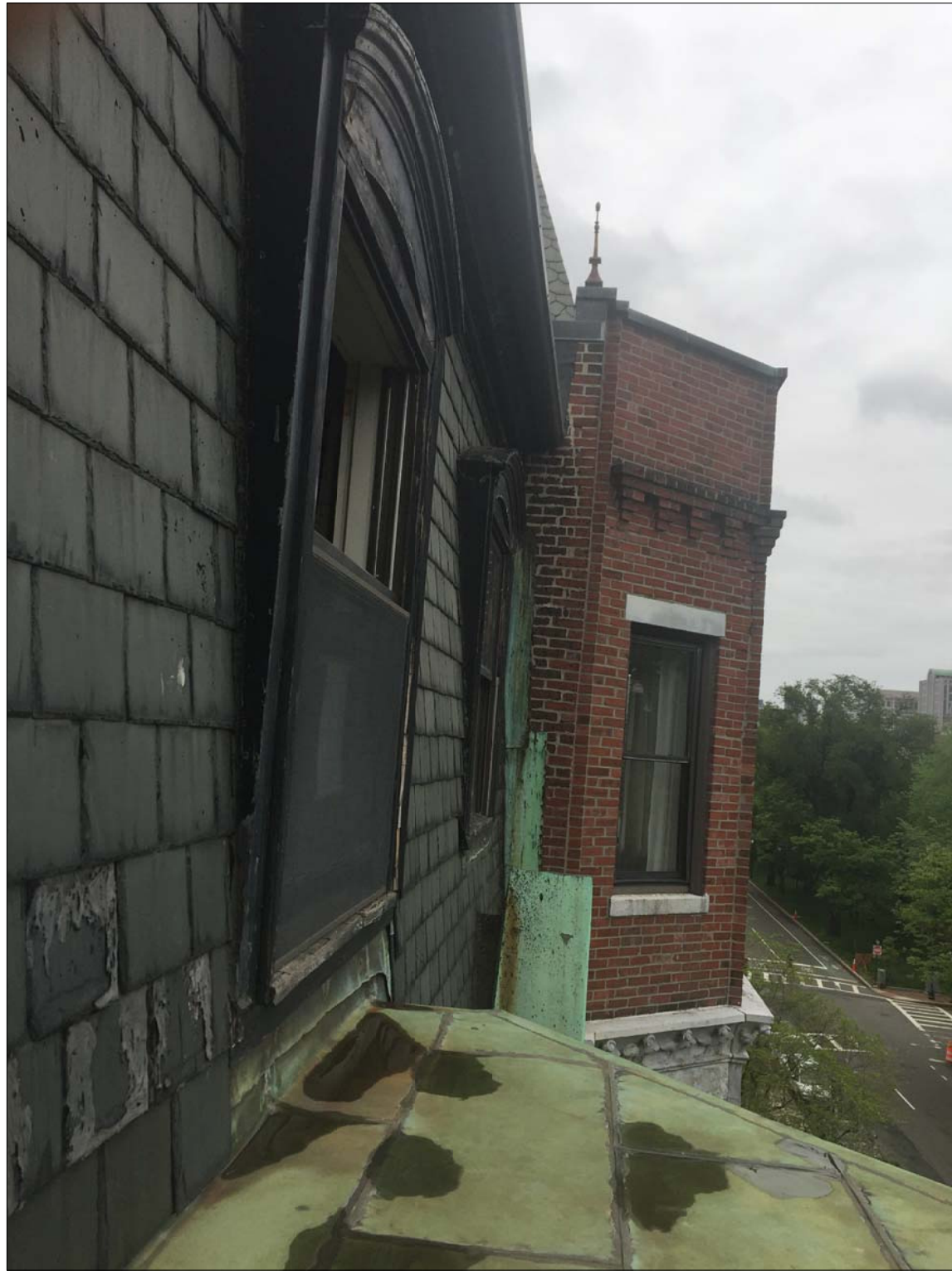
327 COMMONWEALTH AVENUE EXTERIOR BRICK WINDOW
