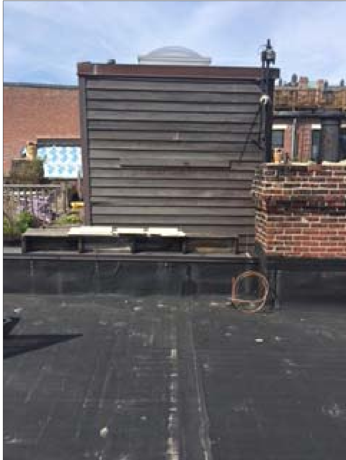
327 COMMONWEALTH AVENUE HEADHOUSE
