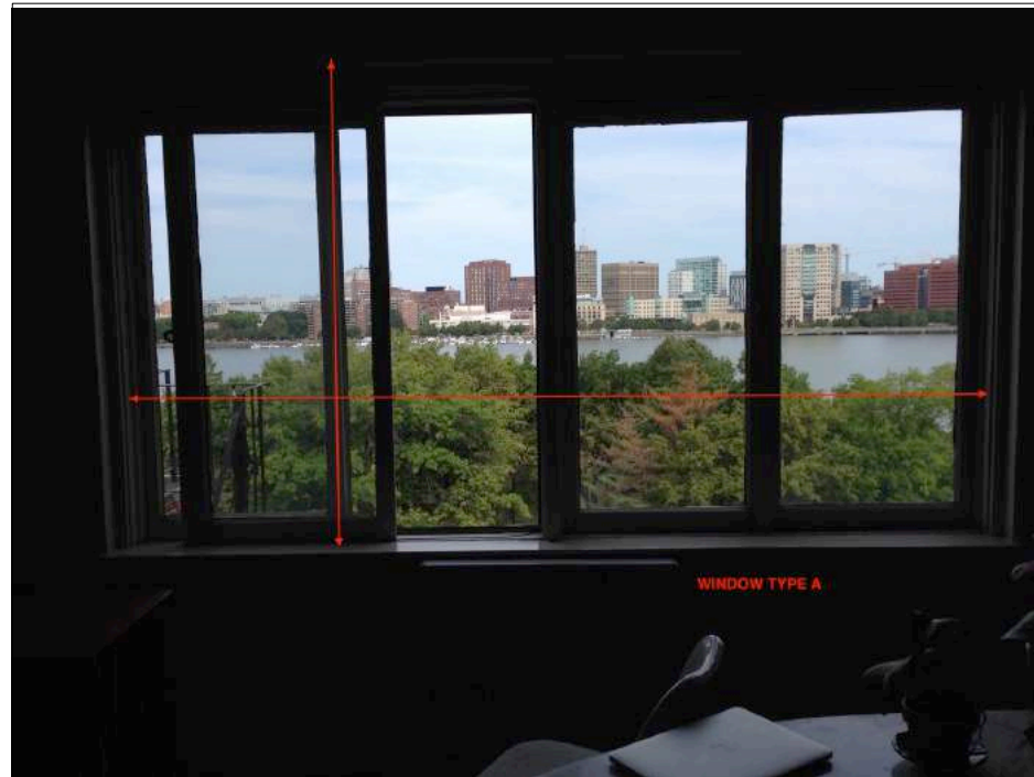
Photo1-Interior View of Existing Window
