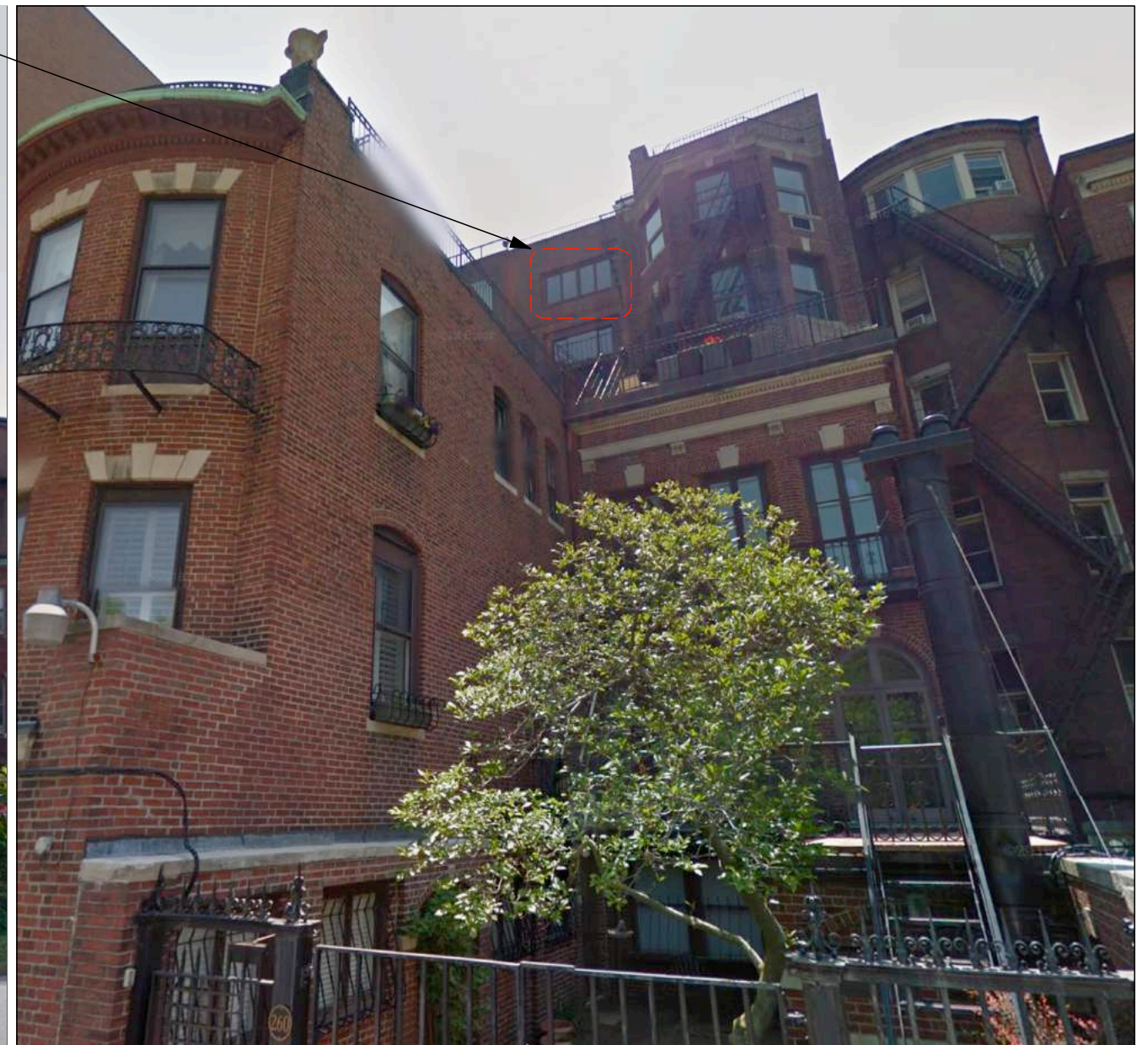
2.Existing Condition View of Rear Elevation
