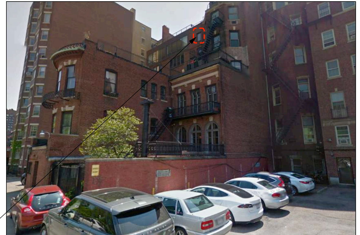
Photo3-Rear Elevation Existing Condition
