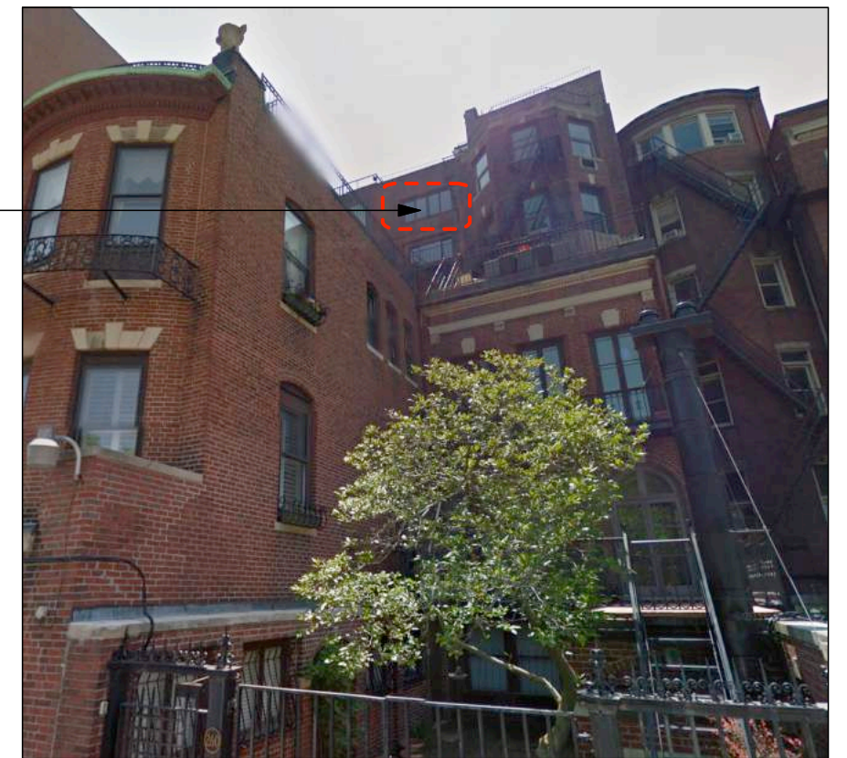
Photo4-Rear Elevation Existing Condition
