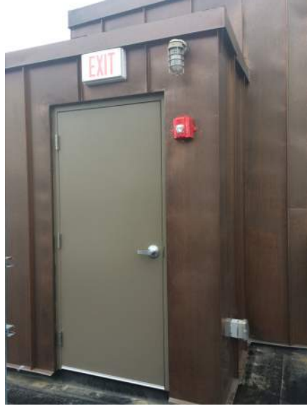
SIMILAR INSTALLED APPLICATION OF COPPER WALL PANELS
