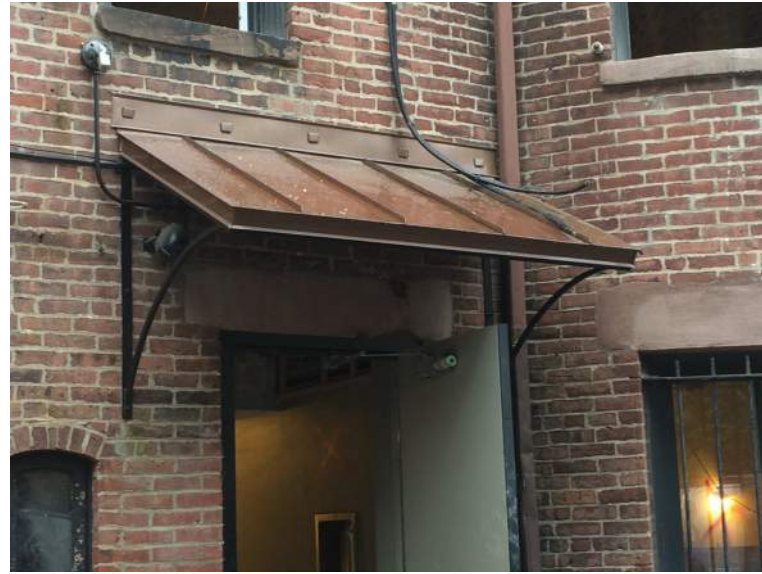
SIMILAR INSTALLED APPLICATION OF COPPER CANOPY AND BRACKETS
