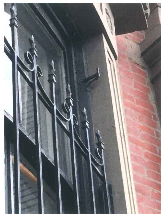
-23- VIEW OF EXISTING DETAILS
