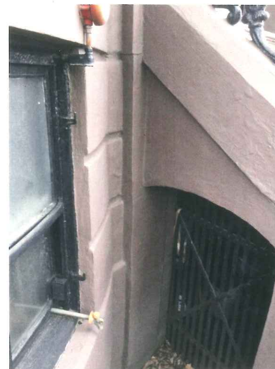
-22- VIEW OF EXISTING DETAILS
