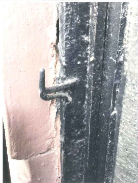
-21- VIEW OF EXISTING DETAILS
