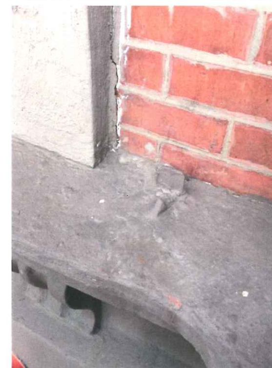
-24- VIEW OF EXISTING DETAILS
