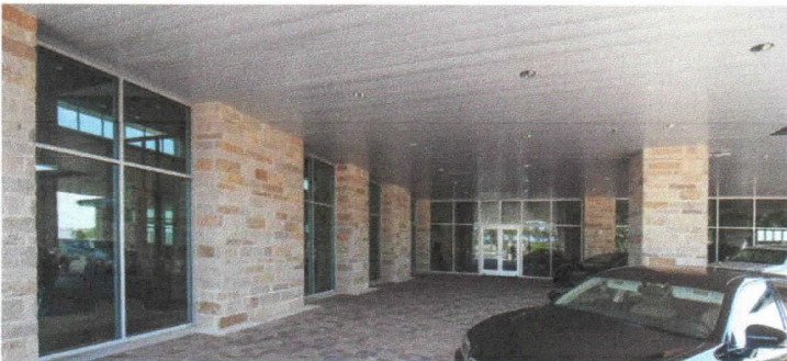
Berridge L-Panel is a great soffit panel and can be site-formed with the FP-16 portable roll former.
