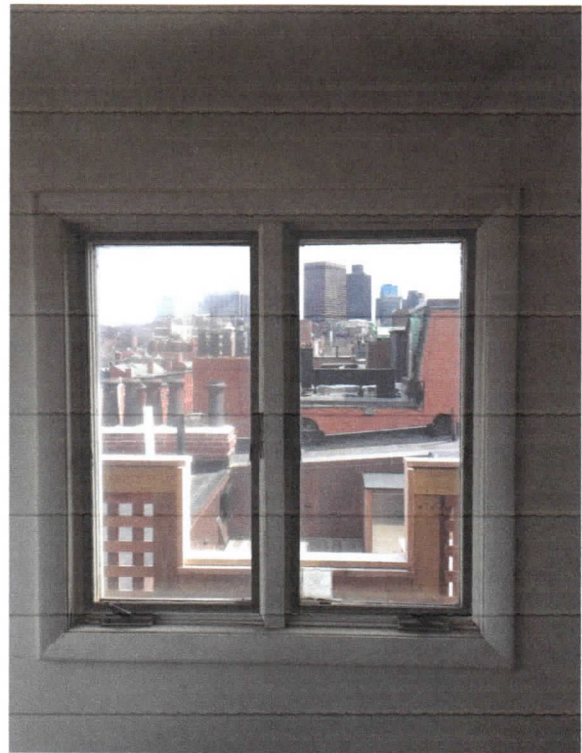
Side, Casement Window East Exposure
