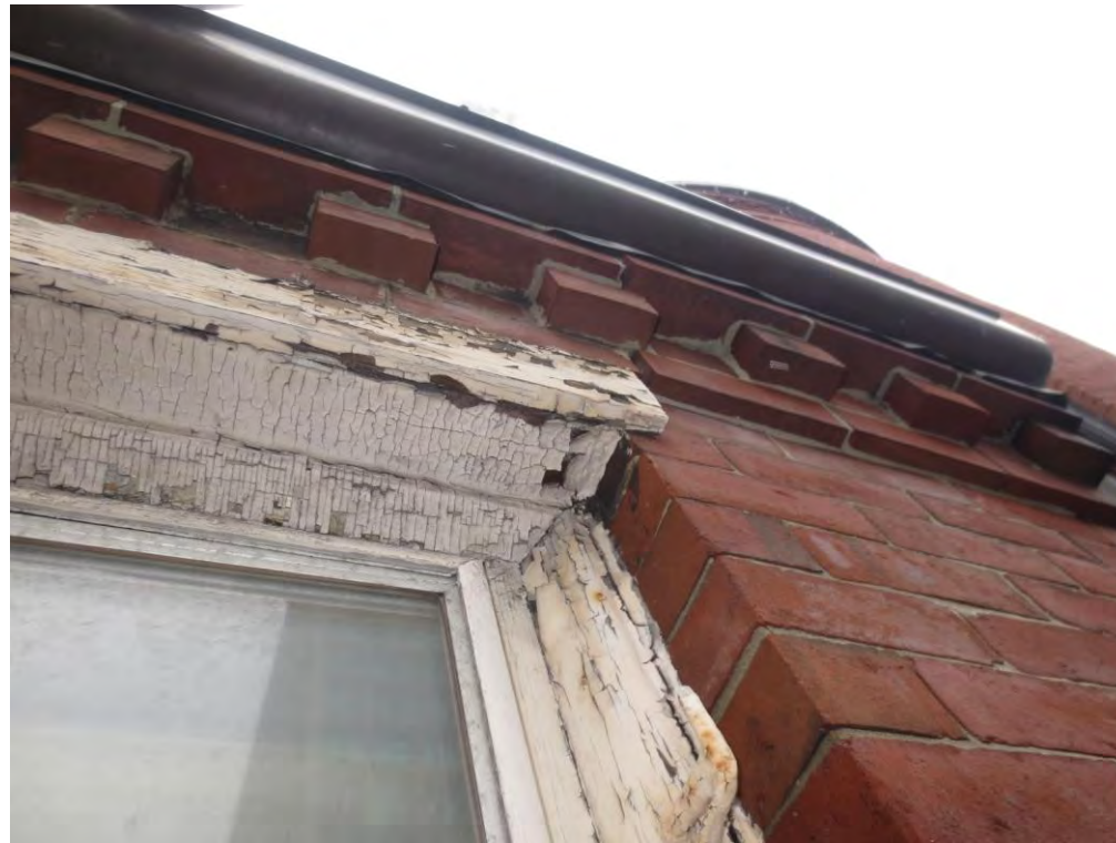
Wood Lintel at Fourth Floor Front Window
