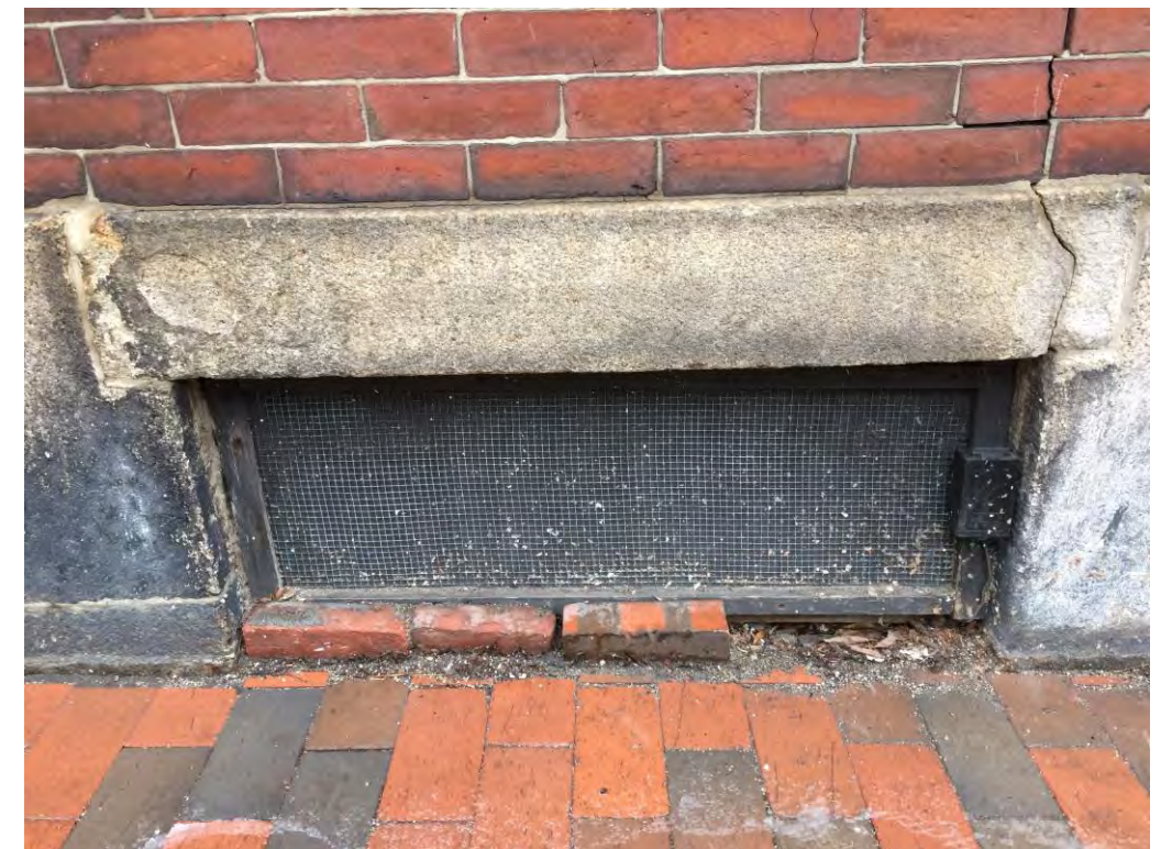
Basement Opening (Right)
