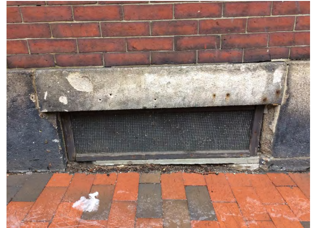
Basement Opening (Left) with Concrete Sill
