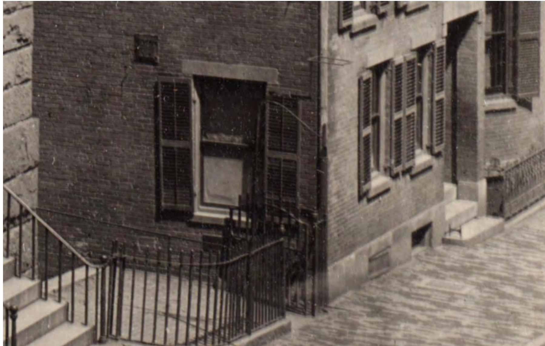
Historic photo showing basement openings Historic New England Nathaniel Stebbins Collection (1847-1922) Reference code PC047.02.6120.NN004
