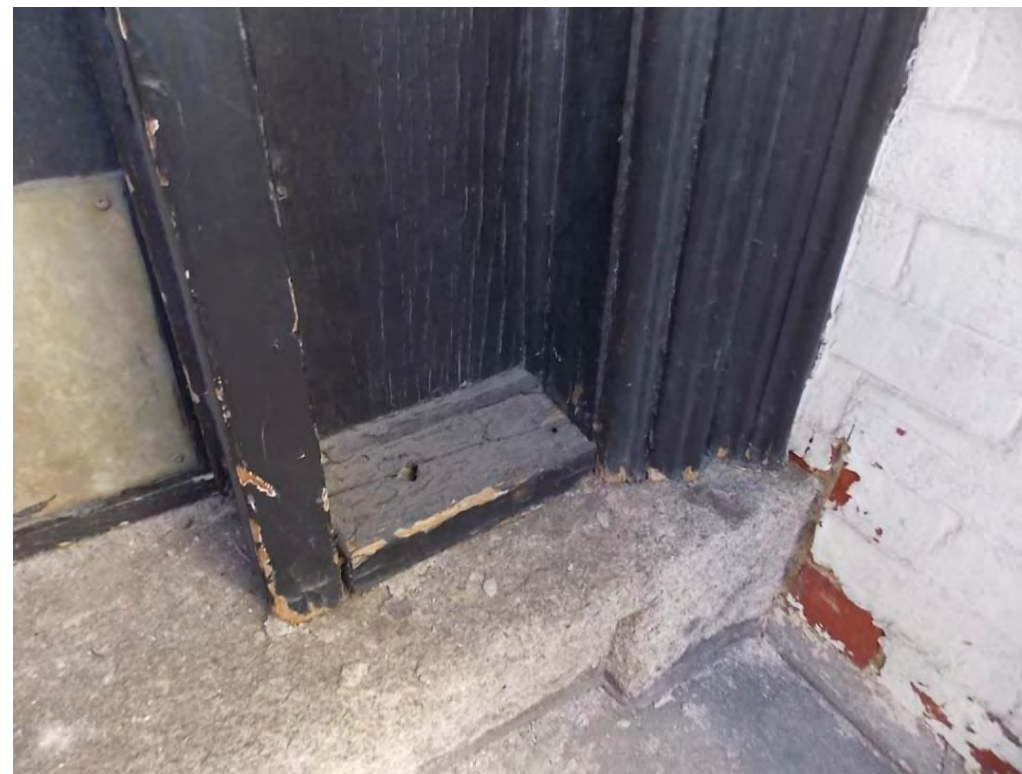
Front Door Detail
