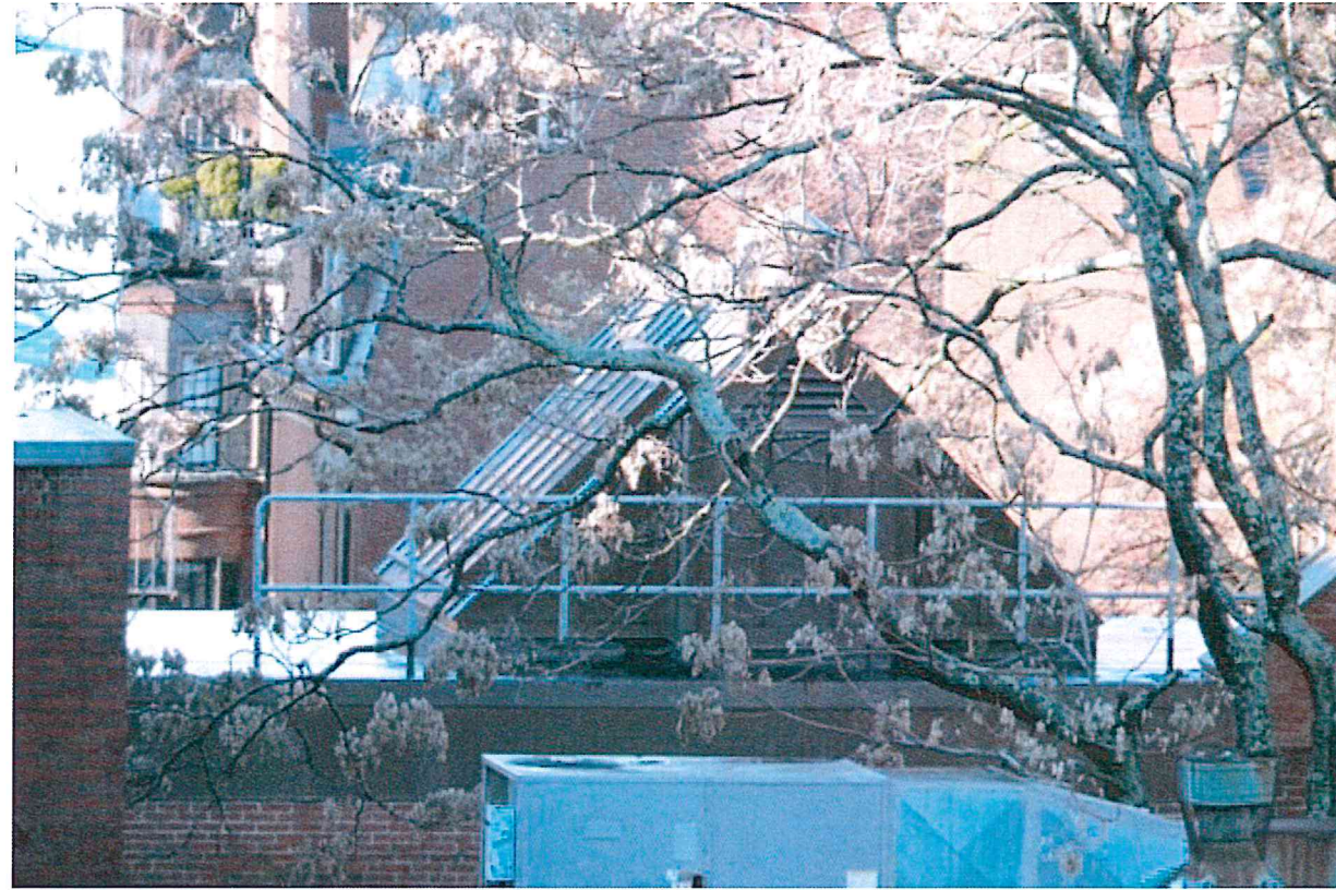
IMAGE 2: 42 BEACON STREET ROOF STRUCTURE
