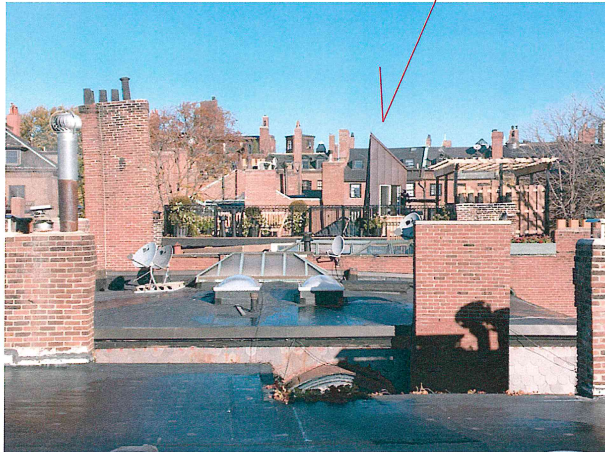
IMAGE 1: VIEW OF 10 WALNUT STREET ROOF STRUCTURE
