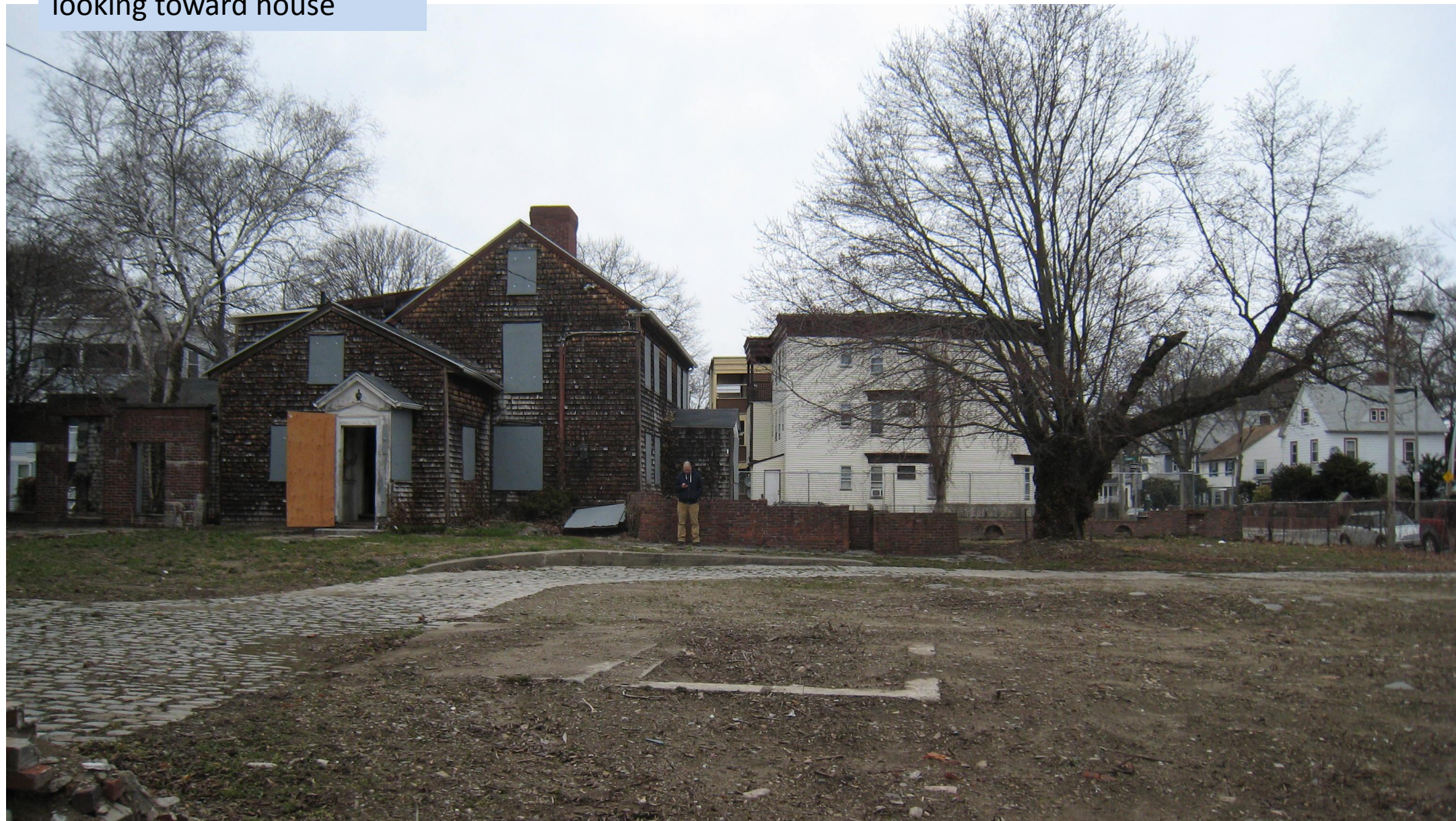
Current view from here looking toward house
