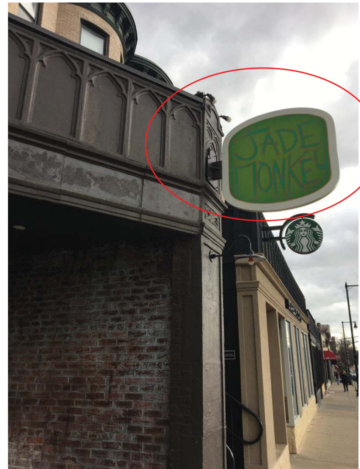
AFTER MARCH 2017 – 1952 Beacon Street
