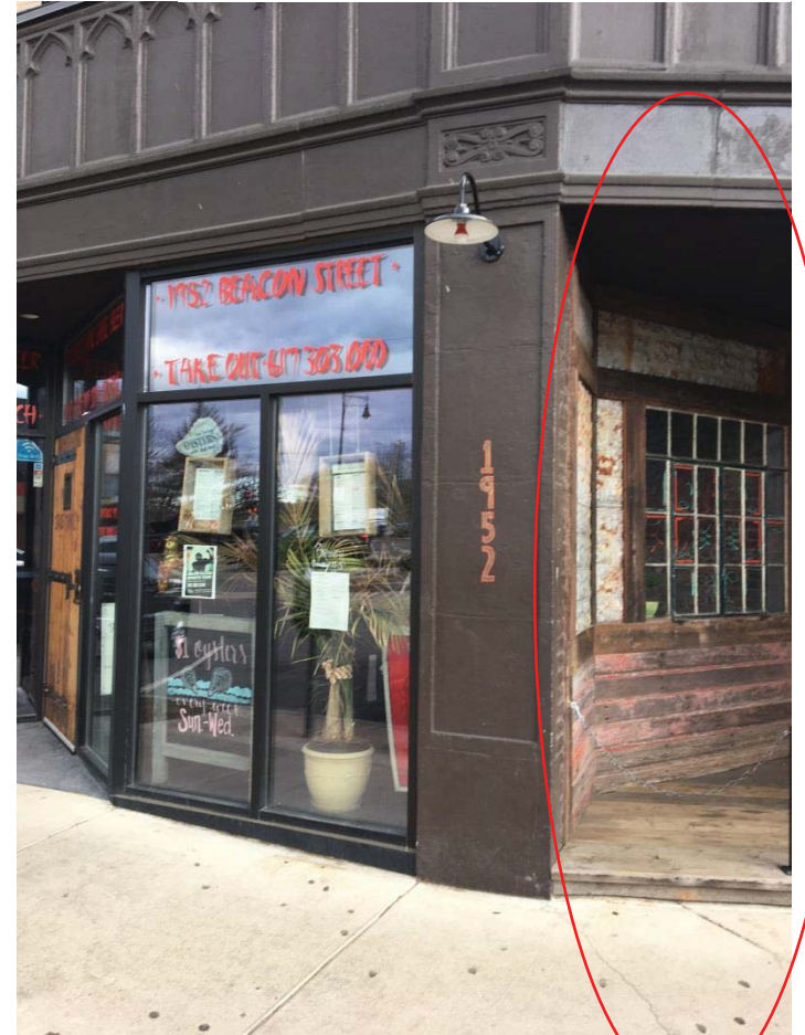
AFTER MARCH 2017 – 1952 Beacon Street
