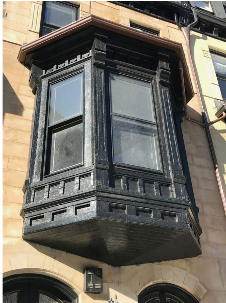
MARLBOROUGH STREET BAY WINDOW
