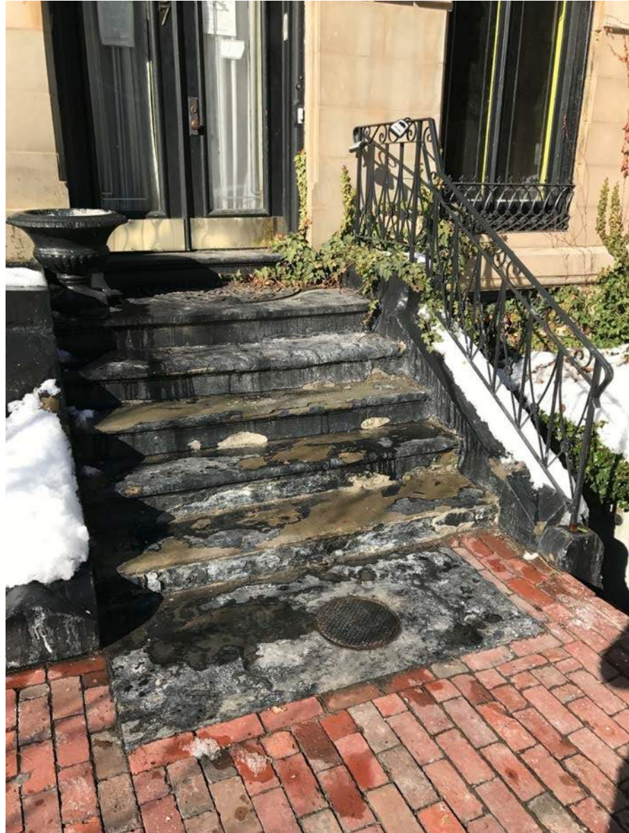
MARLBOROUGH STREET ENTRY WALK
