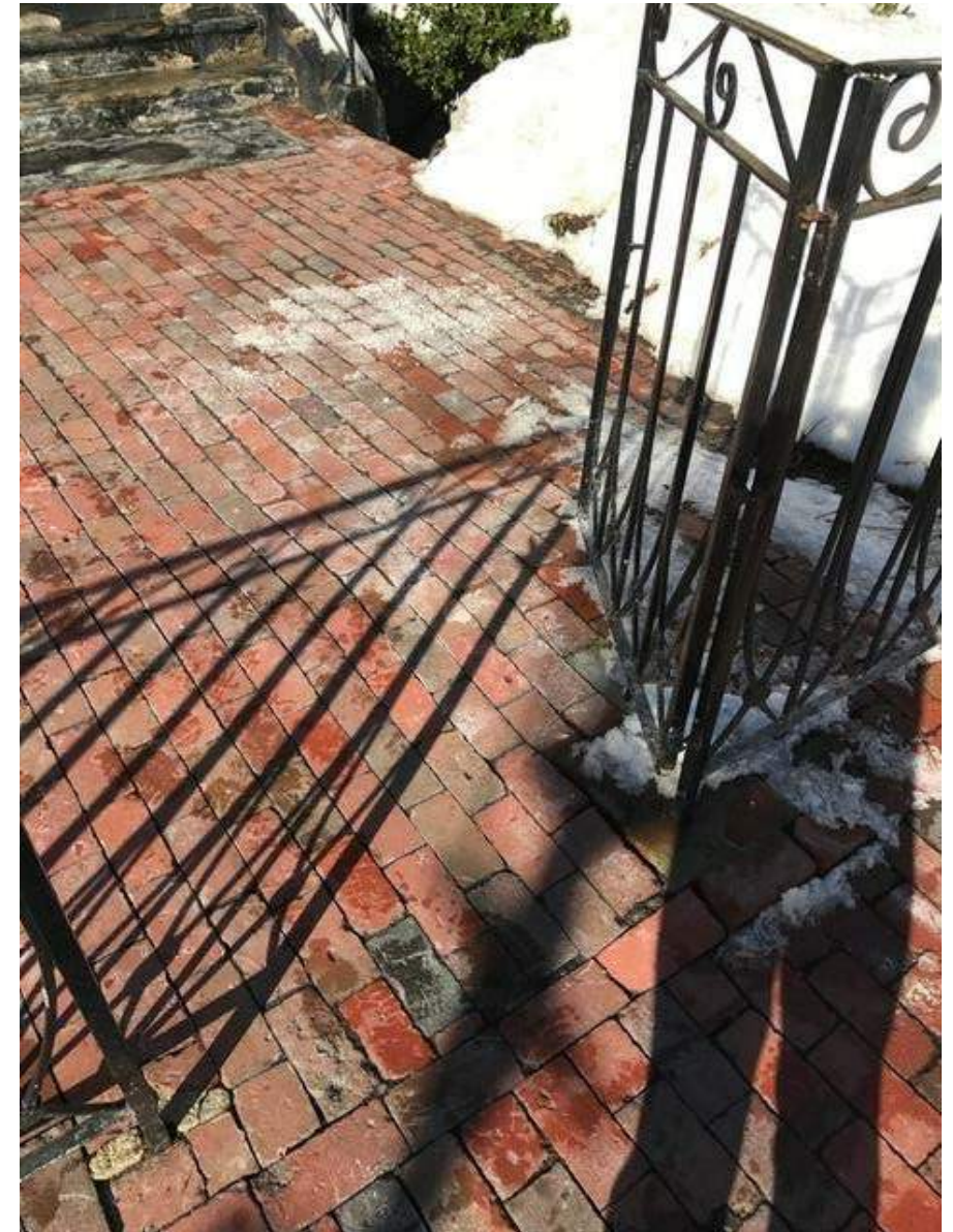
MARLBOROUGH STREET ENTRY WALK
