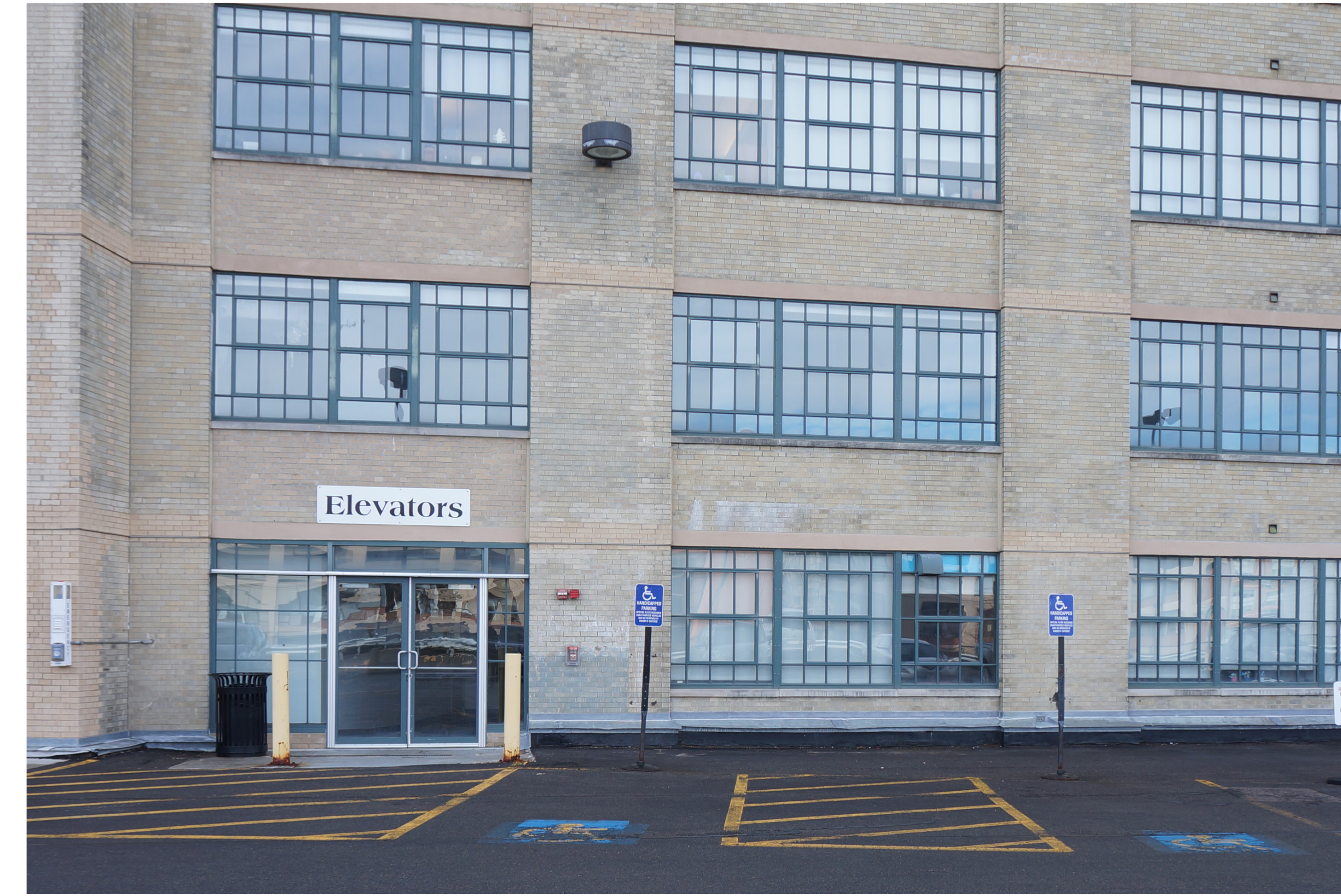
11 LEVEL 4/P6 ENTRANCE FROM PARKING
