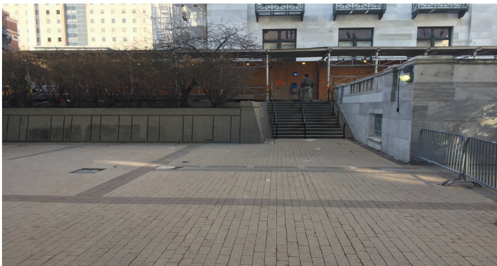
Ramp C: Existing Conditions (3) (Left)
