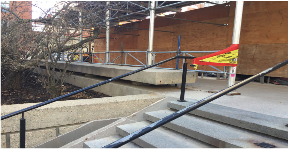
Ramp C: Existing Conditions (1) (Left)
