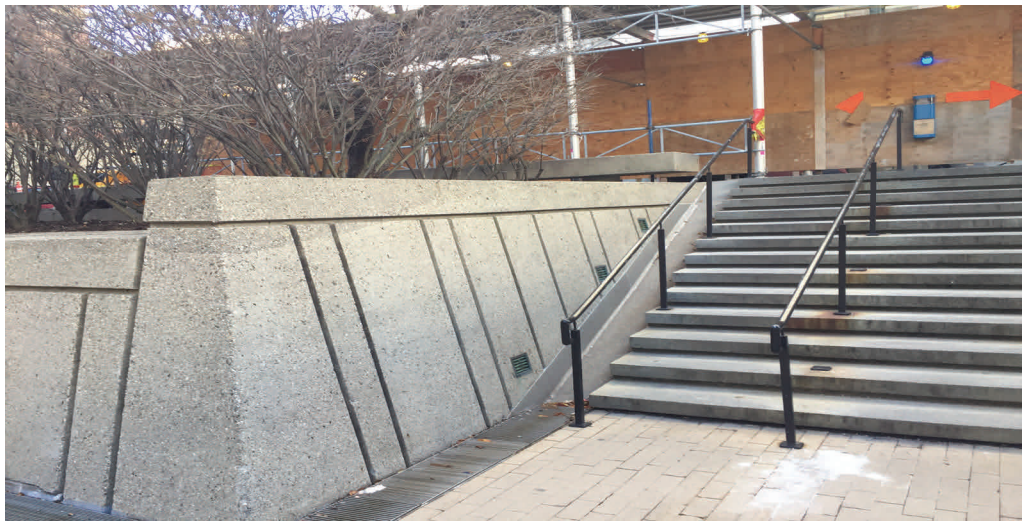
Ramp C: Existing Conditions (2) (Right)
