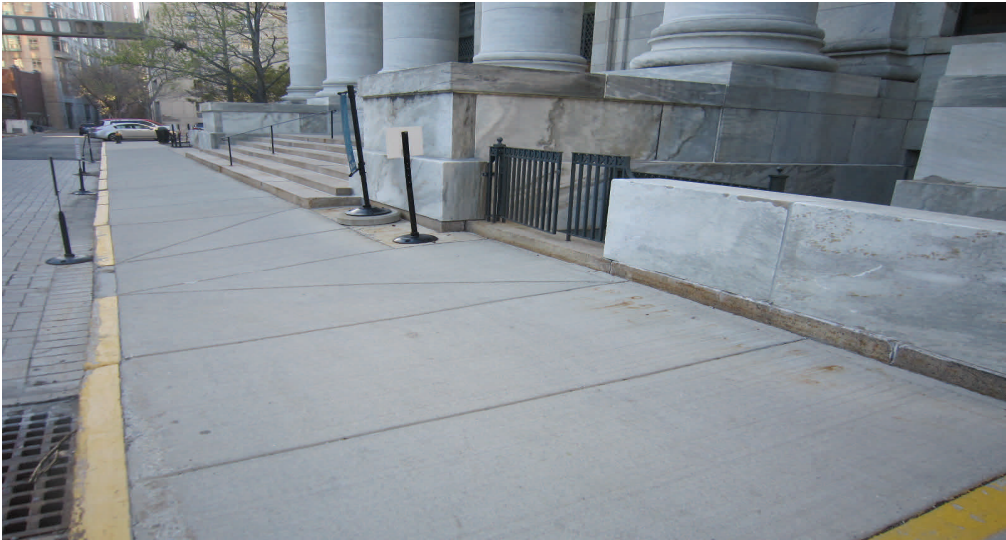
Ramp B: Existing Conditions (2) (Right)
