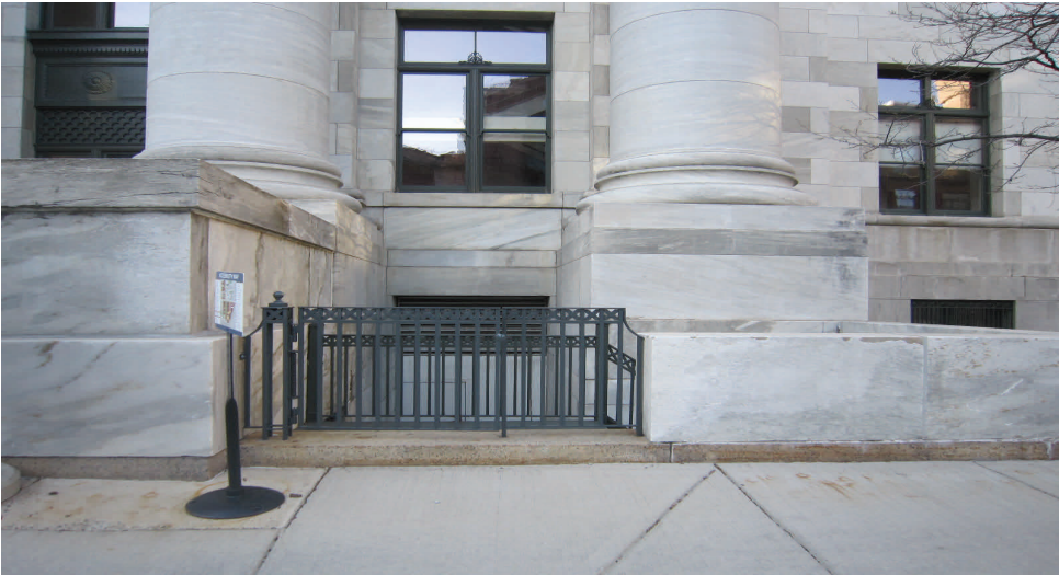
Ramp B: Existing Conditions (1) (Left)
