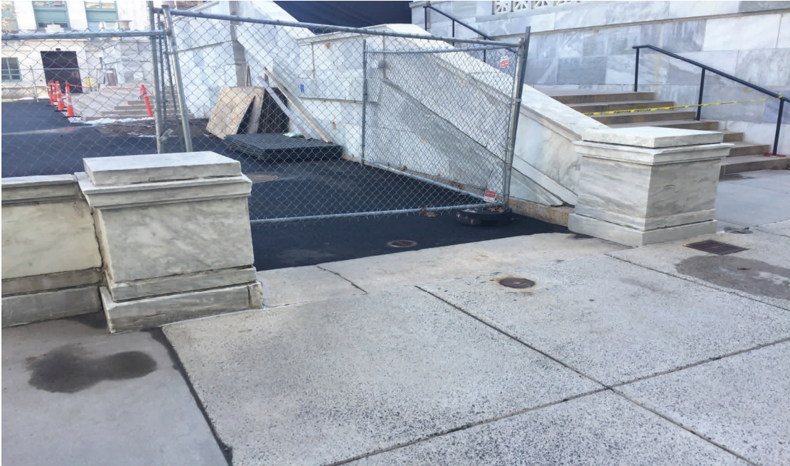
Ramp A: Existing Conditions (1)
