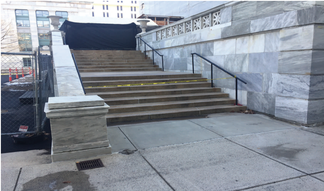
Ramp A: Existing Conditions (2)
