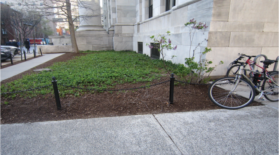
Ramp B: Existing Conditions (3) (Left)
