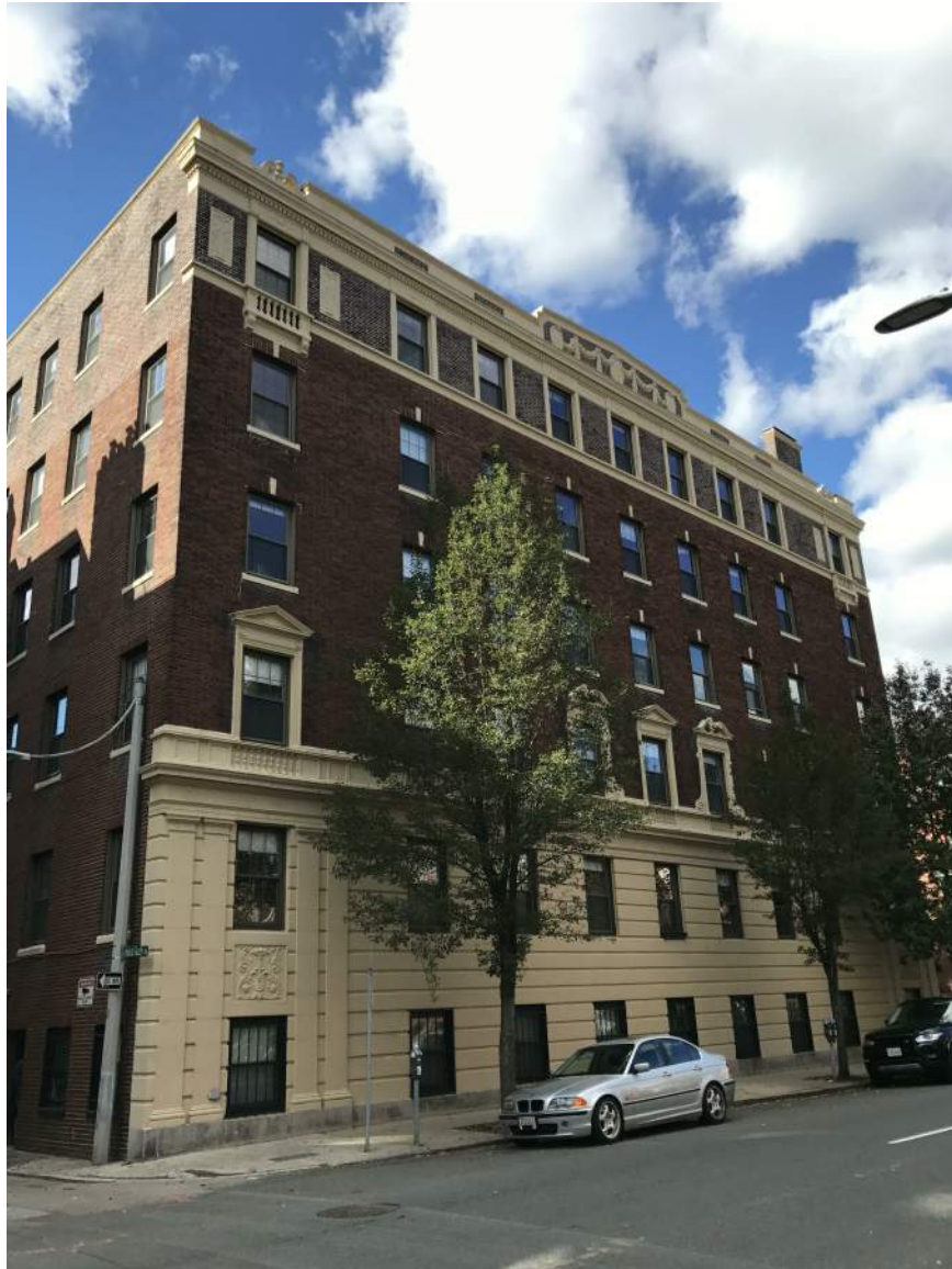
GLOUCESTER STREET FACADE
