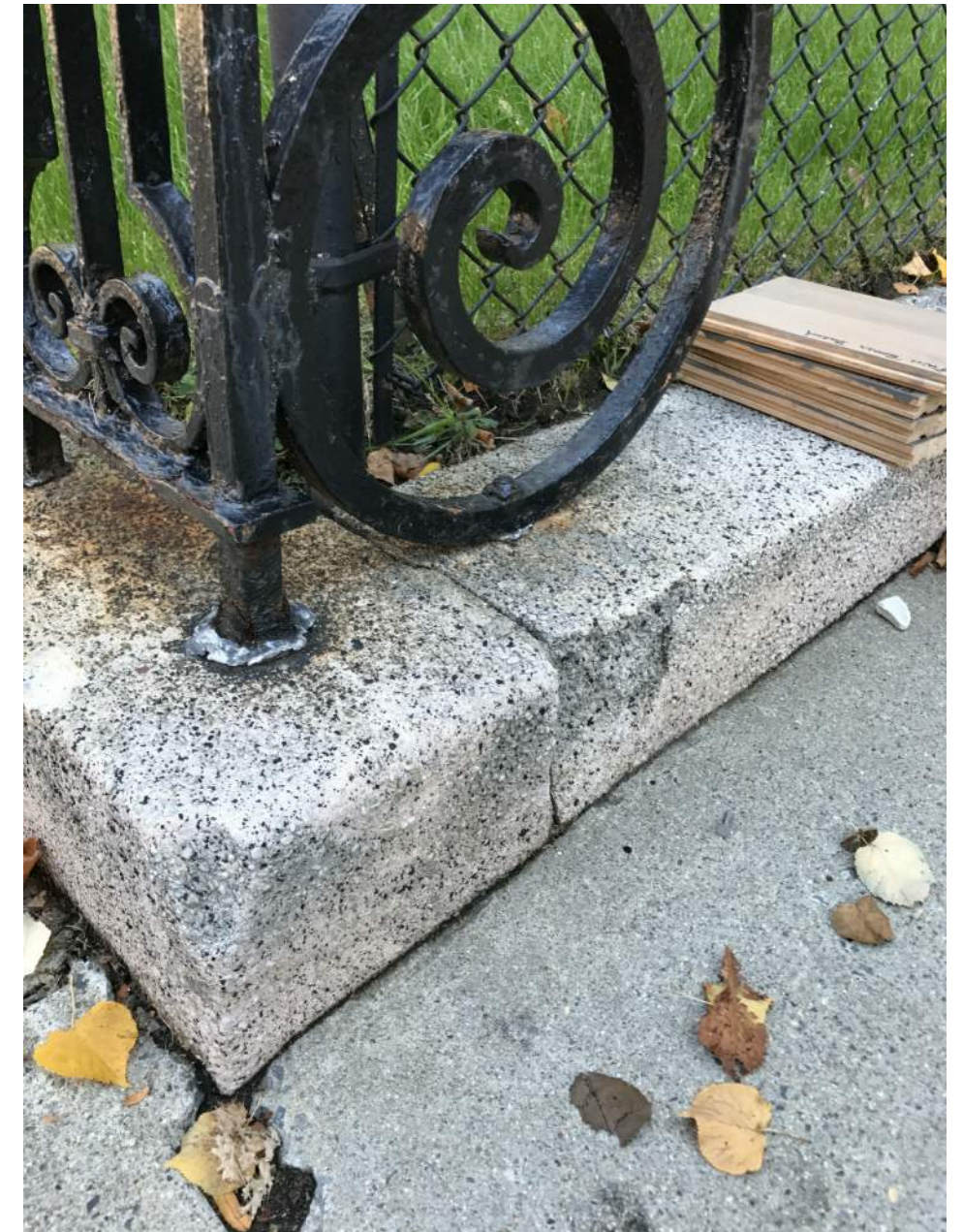
REPAIR, PATCH AND CLEAN EXISTING CONCRETE CURB
