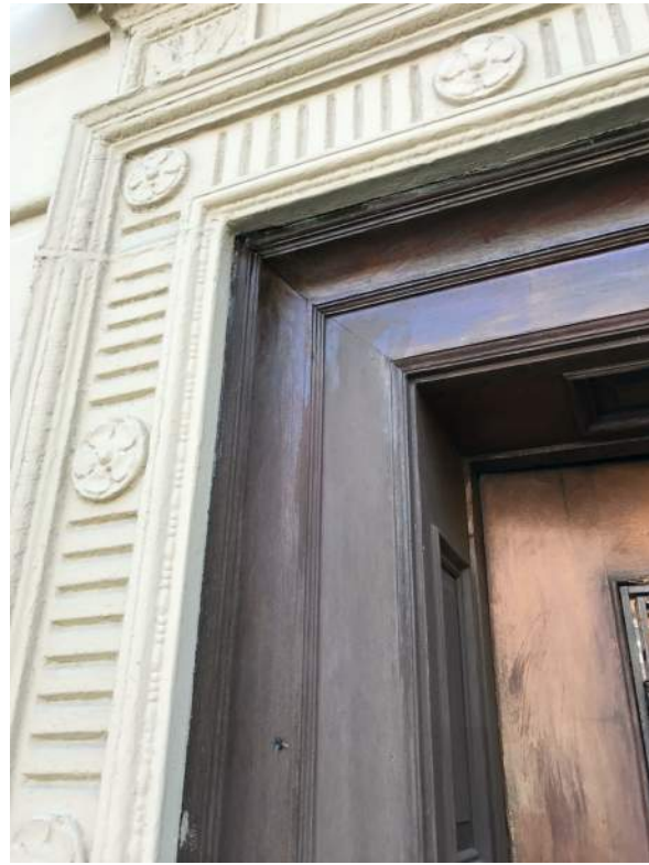
401 BEACON STREET - EXISTING DOOR AND SURROUND CONDITIONS
