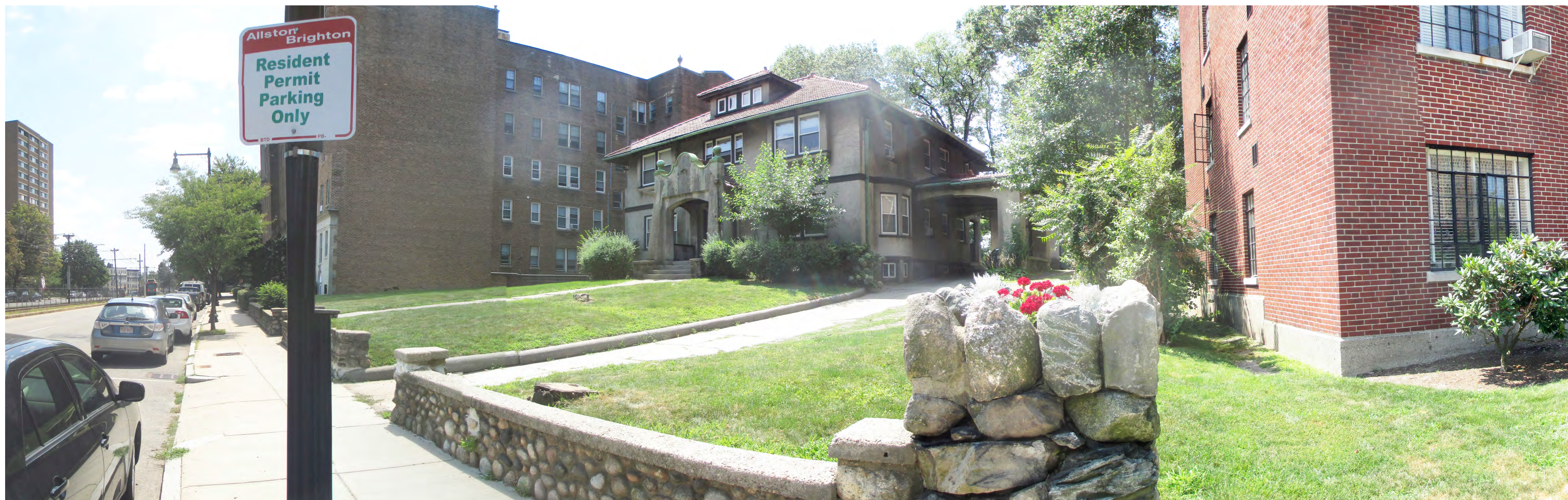
EXISTING SIDE VIEW FROM COMMONWEALTH AVENUE
