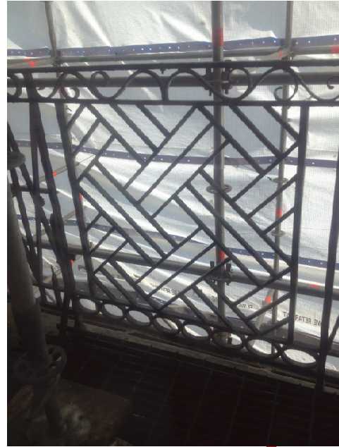
PARTIAL SOUTH RAILING
