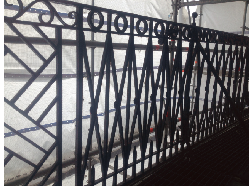
PARTIAL SOUTH RAILING
