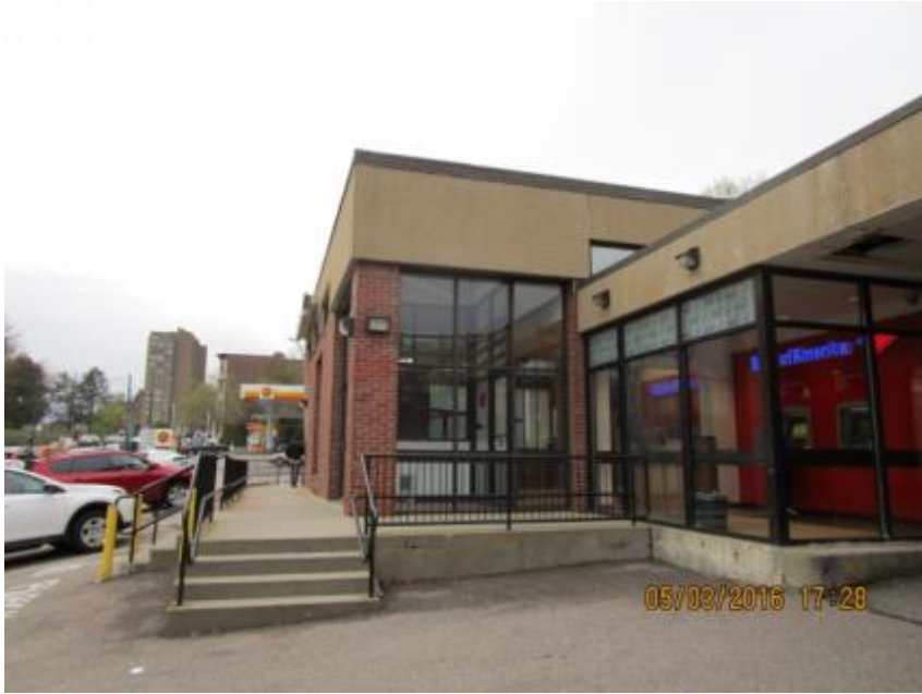
Subject Site – Right elevation May 3, 2016
