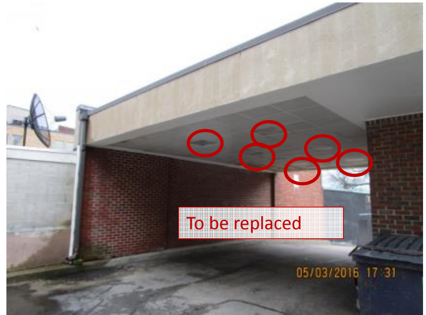
Subject Site – Canopy drive-through May 3, 2016
