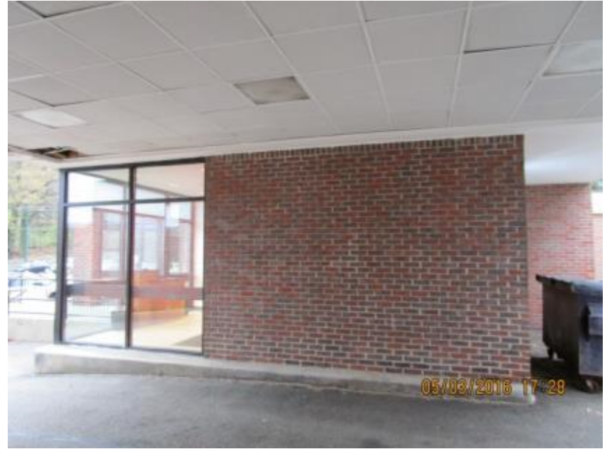
Subject Site – Right elevation May 3, 2016
