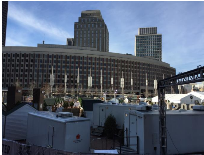
Challenge Temporary utilities and structures clog and damage the Plaza
