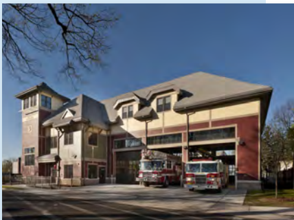
White Street Fire Station Springfield, MA
