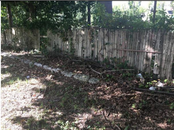
Photo 11: View of a foundation wall on Site Nos. 8 & 9.
