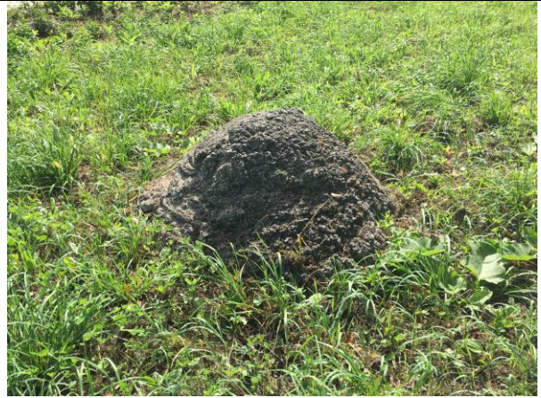
Photo 8: View of concrete dumped on Site No. 15.
