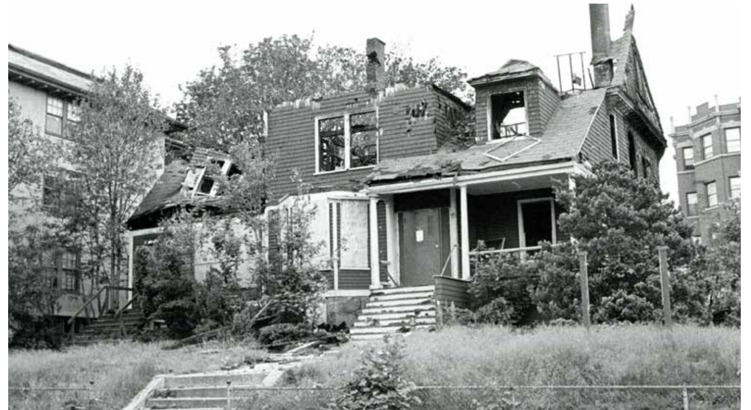
Demolition of former house at 405 Washington Street
